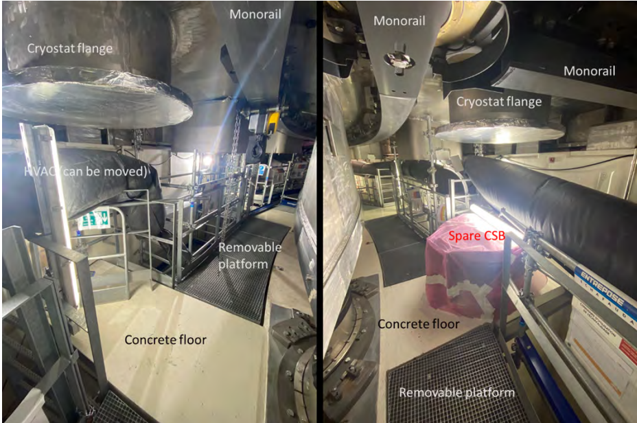
Figure 1 - Left: crown cell environment in the configuration without spare CSB. Right: crown cell environment in the configuration with spare CSB
