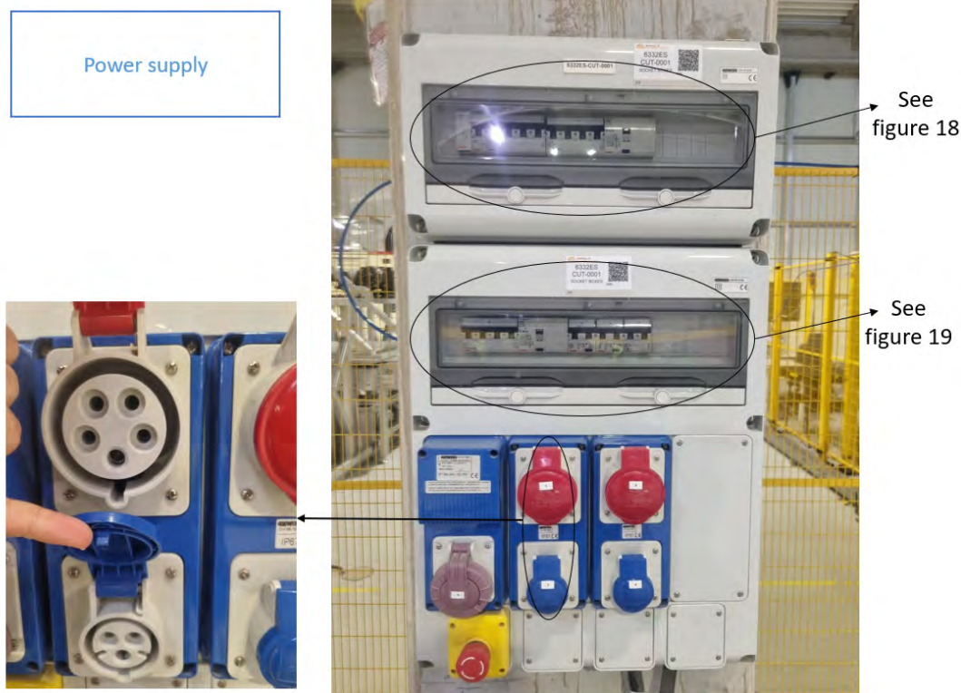
Figure 17 Power supply 32 A – 16 A
