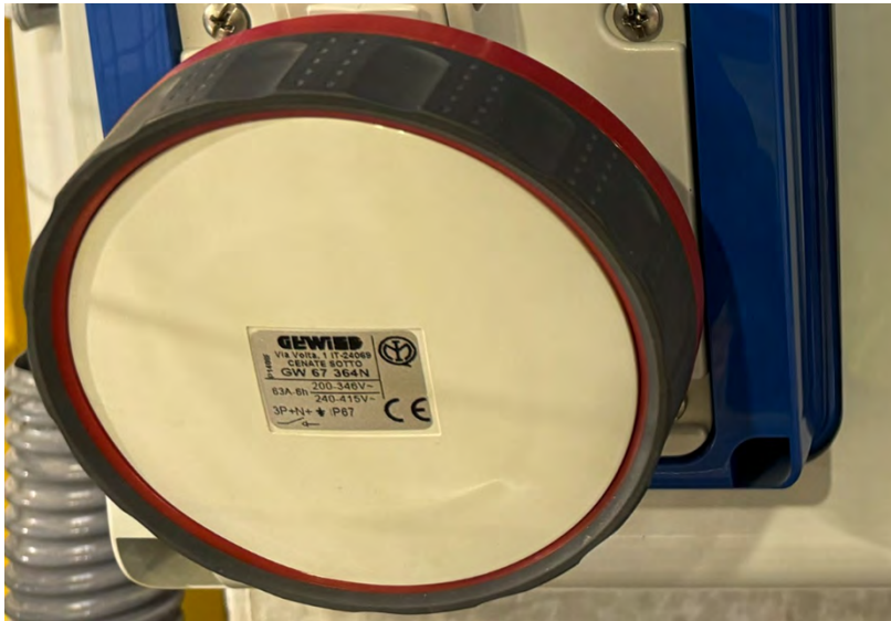
Figure 21 Socket power supply 63 A
