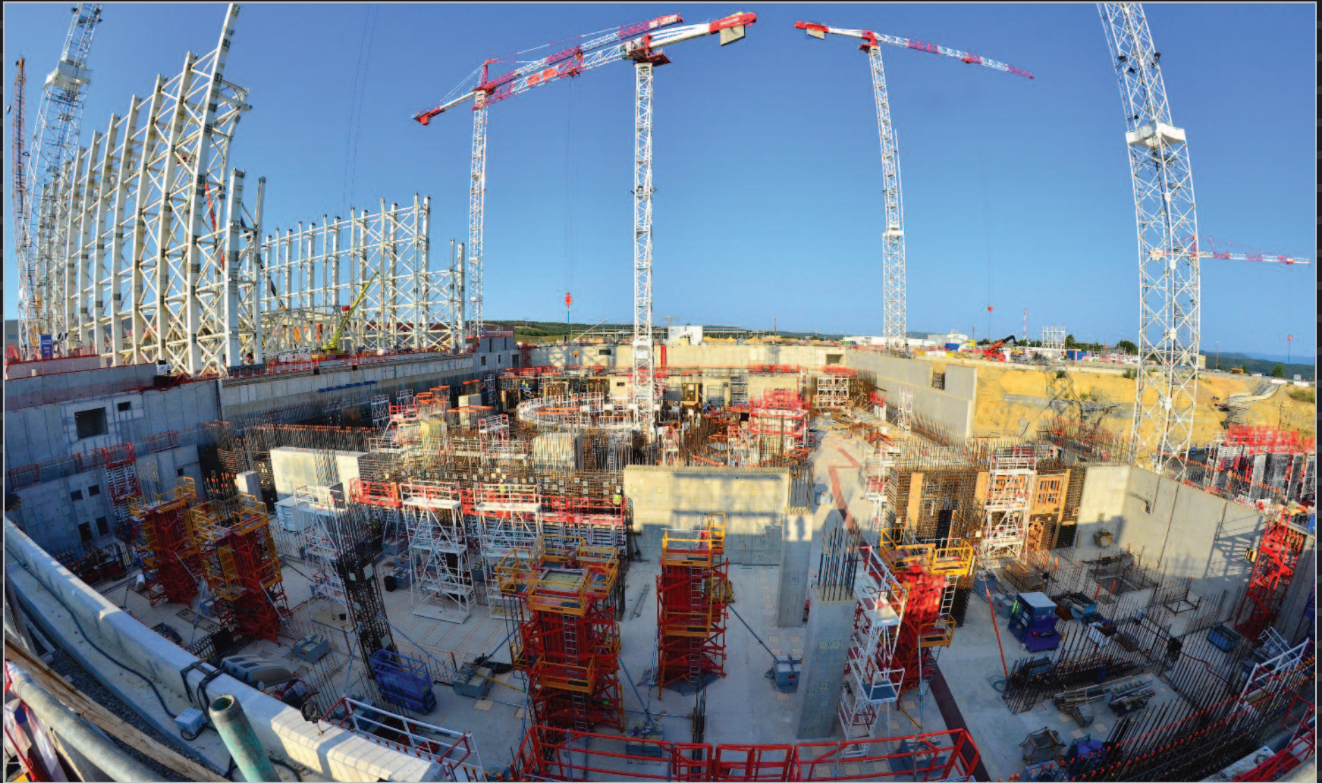
Work progresses in 2015 on the columns and walls of the first basement level (B2) of the Tokamak Complex. At the same time, the metal structure of the giant Assembly Hall takes shape. July 2015
