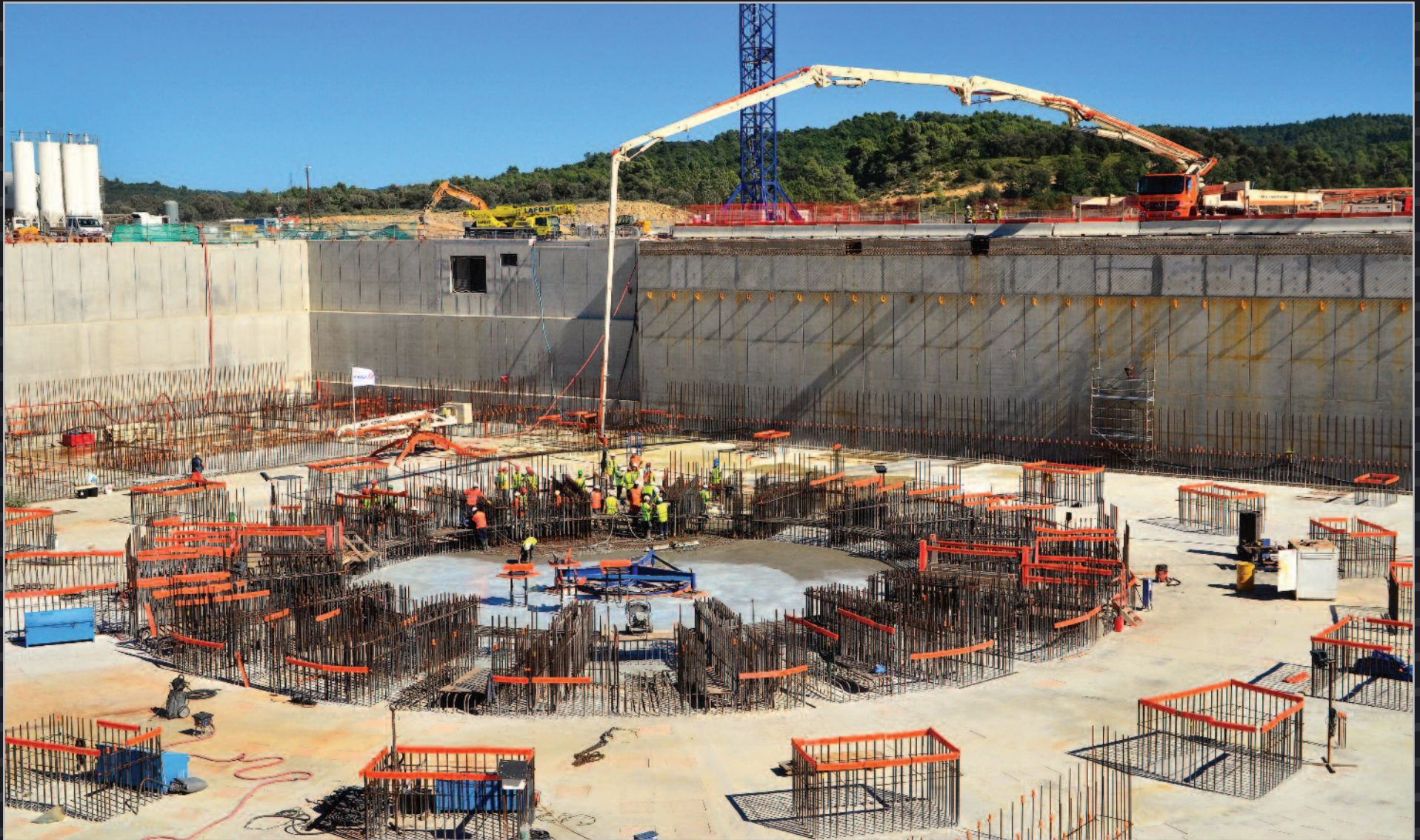
Four years of work in the Tokamak Pit to create the ground support structure and foundations of the Tokamak Complex are brought to a successful conclusion as the last segment of the B2 slab – the basemat that will support the machine and systems – is poured. August 2014
