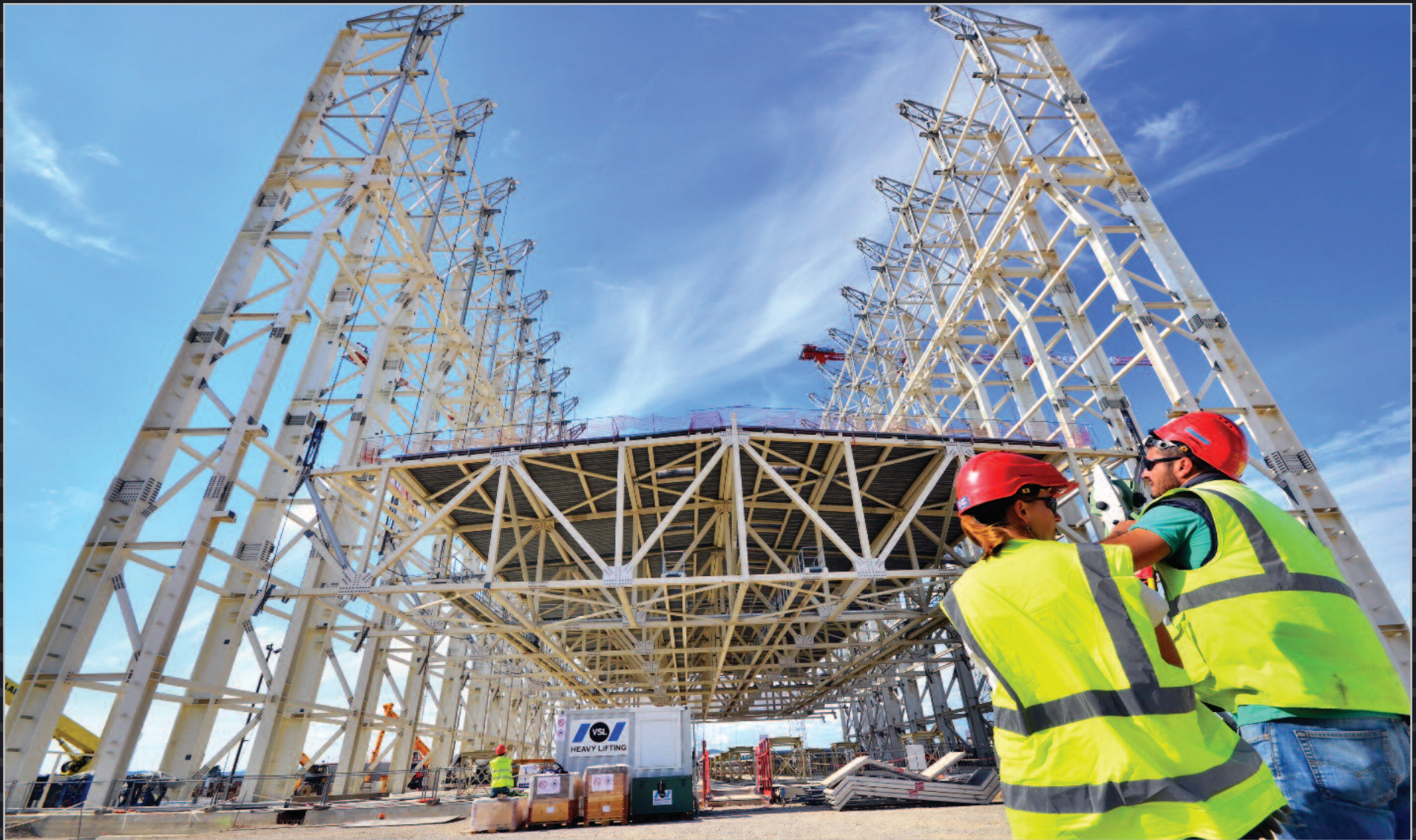
In a carefully programmed operation that lasts 14 hours, the 730-tonne roof structure of the Assembly Building is successfully lifted into place. Now, the building can be fitted out with exterior cladding and rails for the heavy-lift cranes. September 2015
