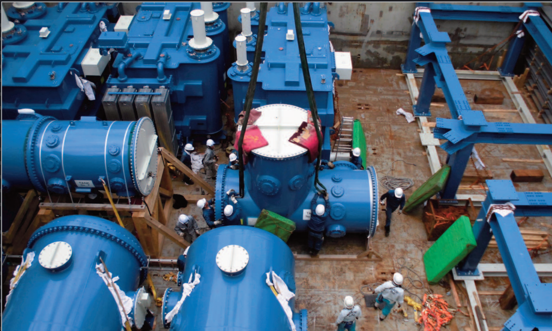
Three DC generators (0.2MV, 0.4MV, 0.6MV), tanks of transmission line 1 & 2, and support frames are transported in the first shipment for the ITER NBTF/Italy. The installation of these components will be started from Dec/2015.
