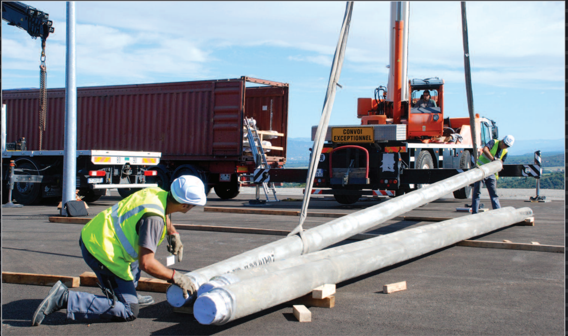
The first cooling water piping under Indian scope reaches ITER in September 2015. In all, India will ship 100 containers of piping for ITER's chilled water and heat rejection systems.
