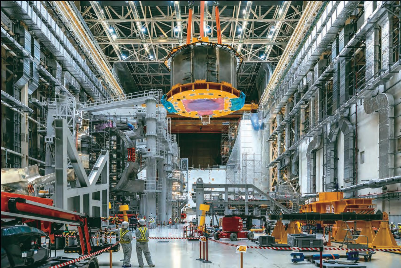
The first of six central solenoid modules is transferred to a staging area in the Assembly Hall. Six modules will be stacked to form the 1,000-tonne central magnet of the ITER machine.
