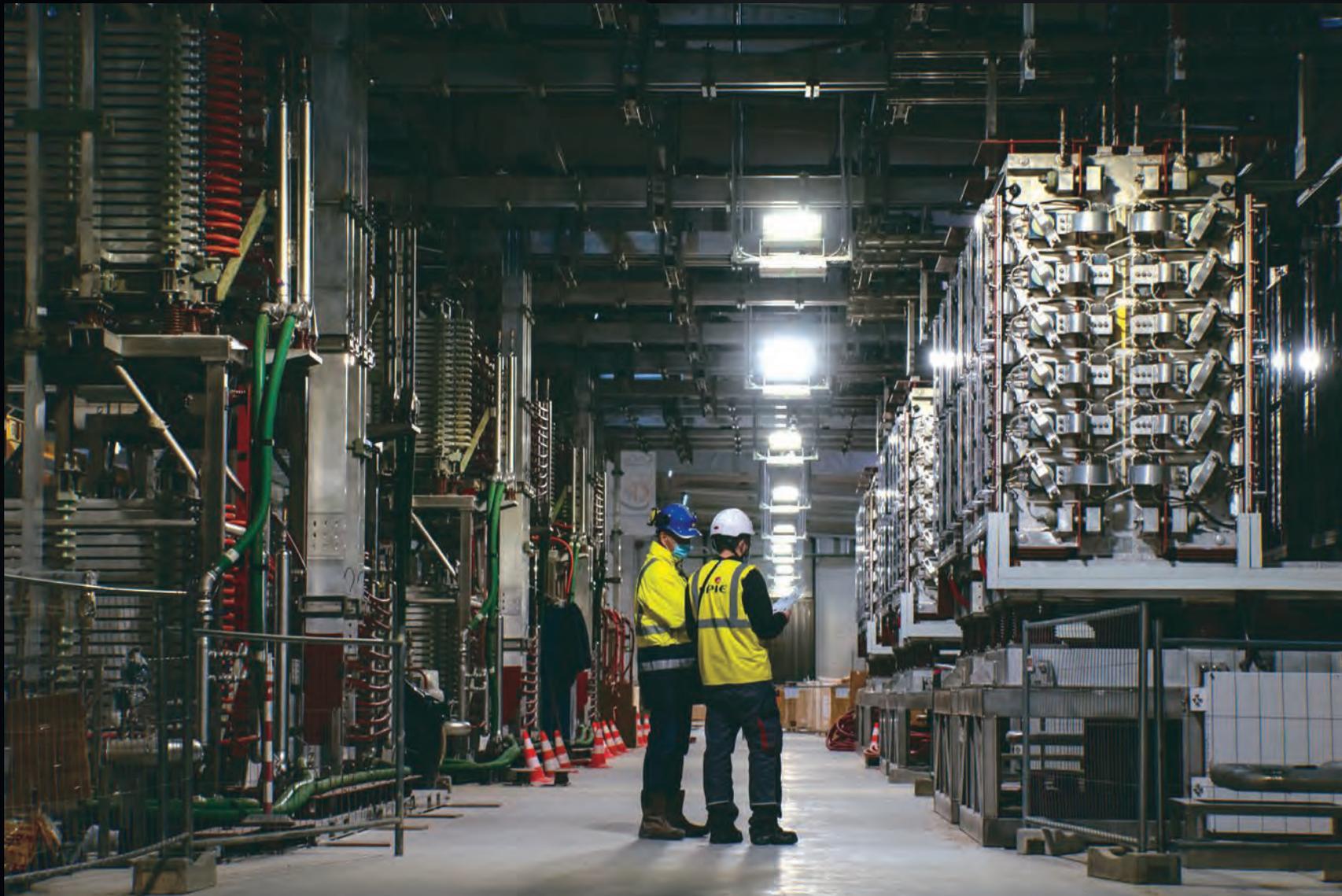
Twin buildings on site are filling up with equipment to convert AC power to DC power for the superconducting magnets. This converter from Korea will be part of equipment that will feed power to the vertical stability coils.
