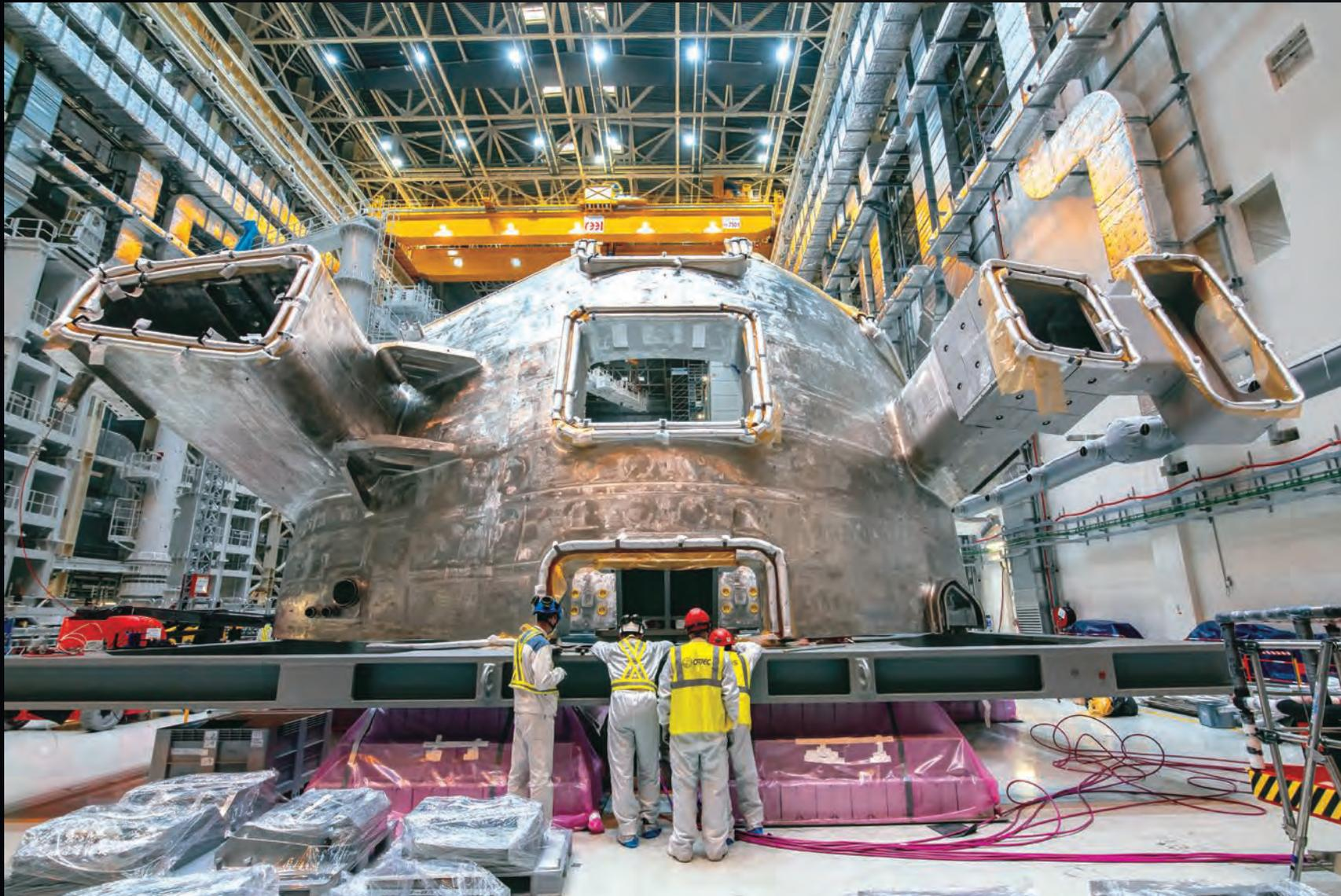
Korea delivers a second vacuum vessel sector to ITER in August 2021. Nine sectors in total will form the torus of the ITER tokamak.
