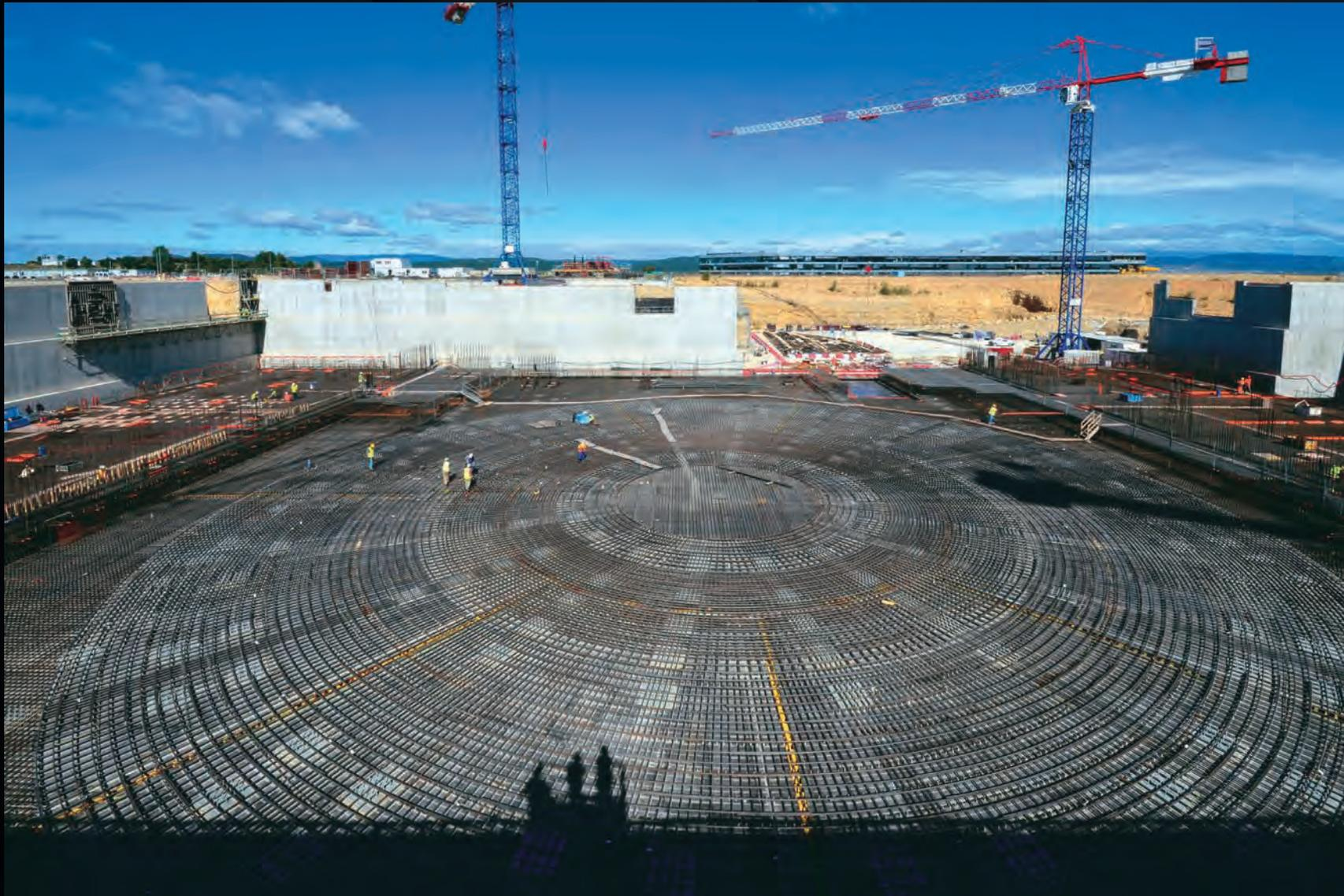
Contractors are preparing to pour 15,000 m<sup>3</sup> of concrete for the "floor" of the Tokamak Complex—the 1.5-metre-thick B2 slab. With rebar, the B2 slab weighs 37,500 tonnes, a load that is supported by 493 seismic pillars.
