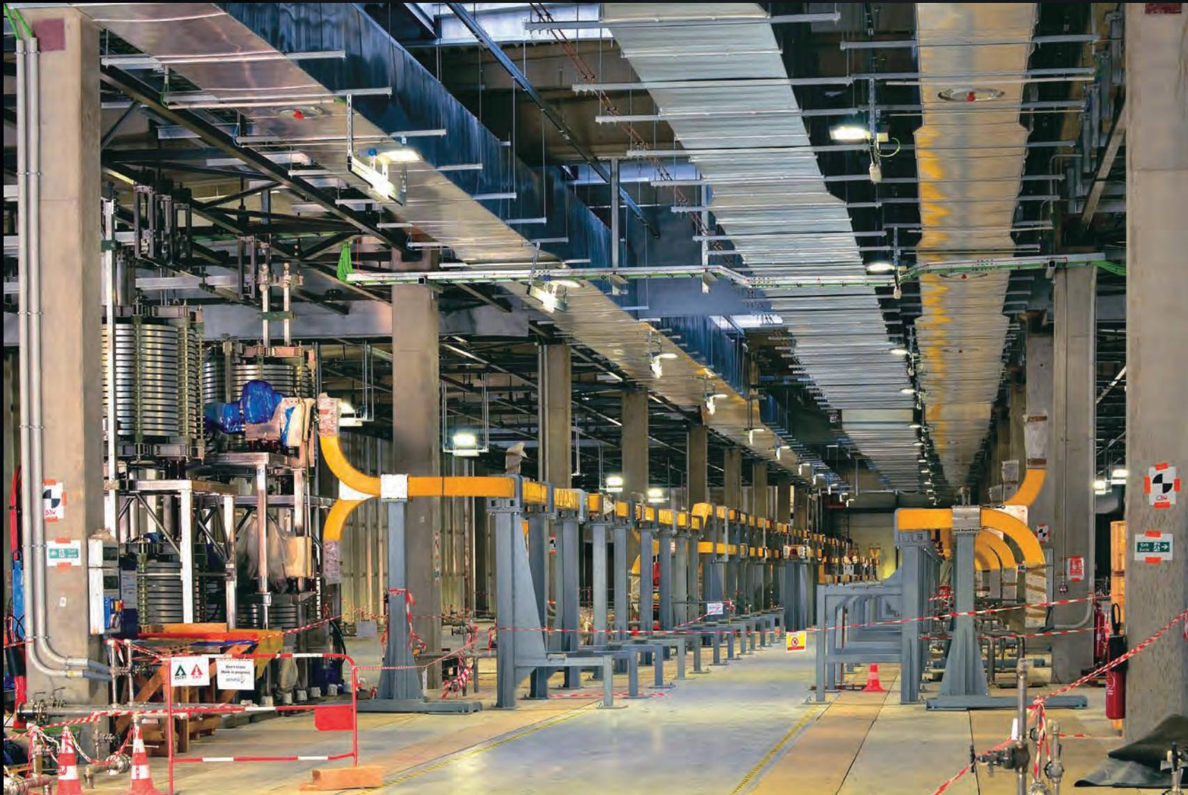
Five kilometres of water-cooled, steel-jacketed busbars will deliver DC power to the ITER magnets. The most powerful will carry close to 70 kiloamps of current—about 7,000 times the power of an average washing machine cable.
