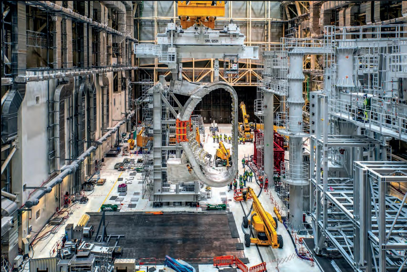
Between the hooks of the overhead crane and the 440-tonne sector module are rigging elements that act as veritable tools, with the capacity to control the load's centre of gravity and pilot the rotation of the component.
