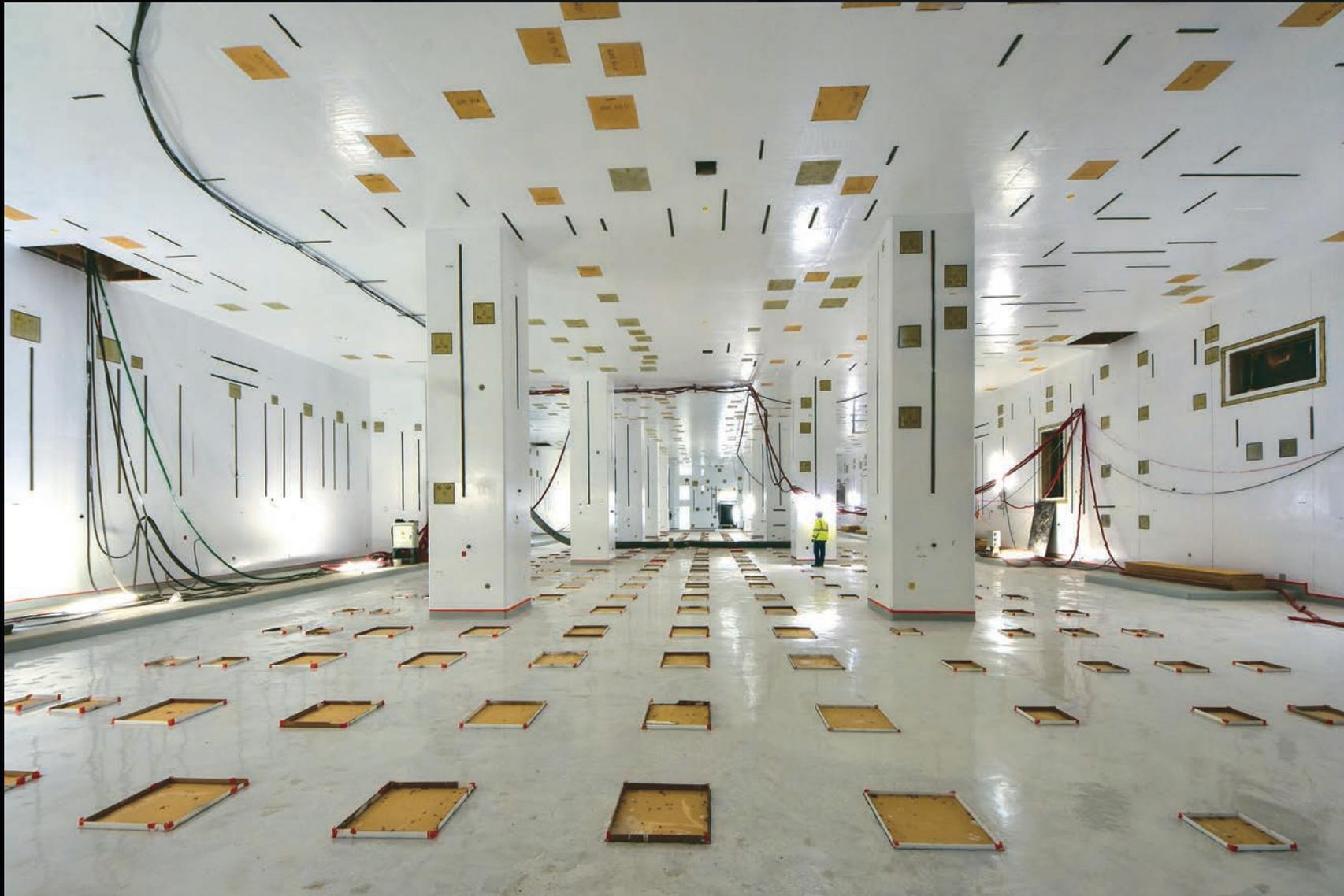
Now painted in white, the lowest basement level of the Diagnostic Building is ready for handover to contractors for the beginning of systems installation. Embedded plates—for the attachment of system supports—are visible on all surfaces.
