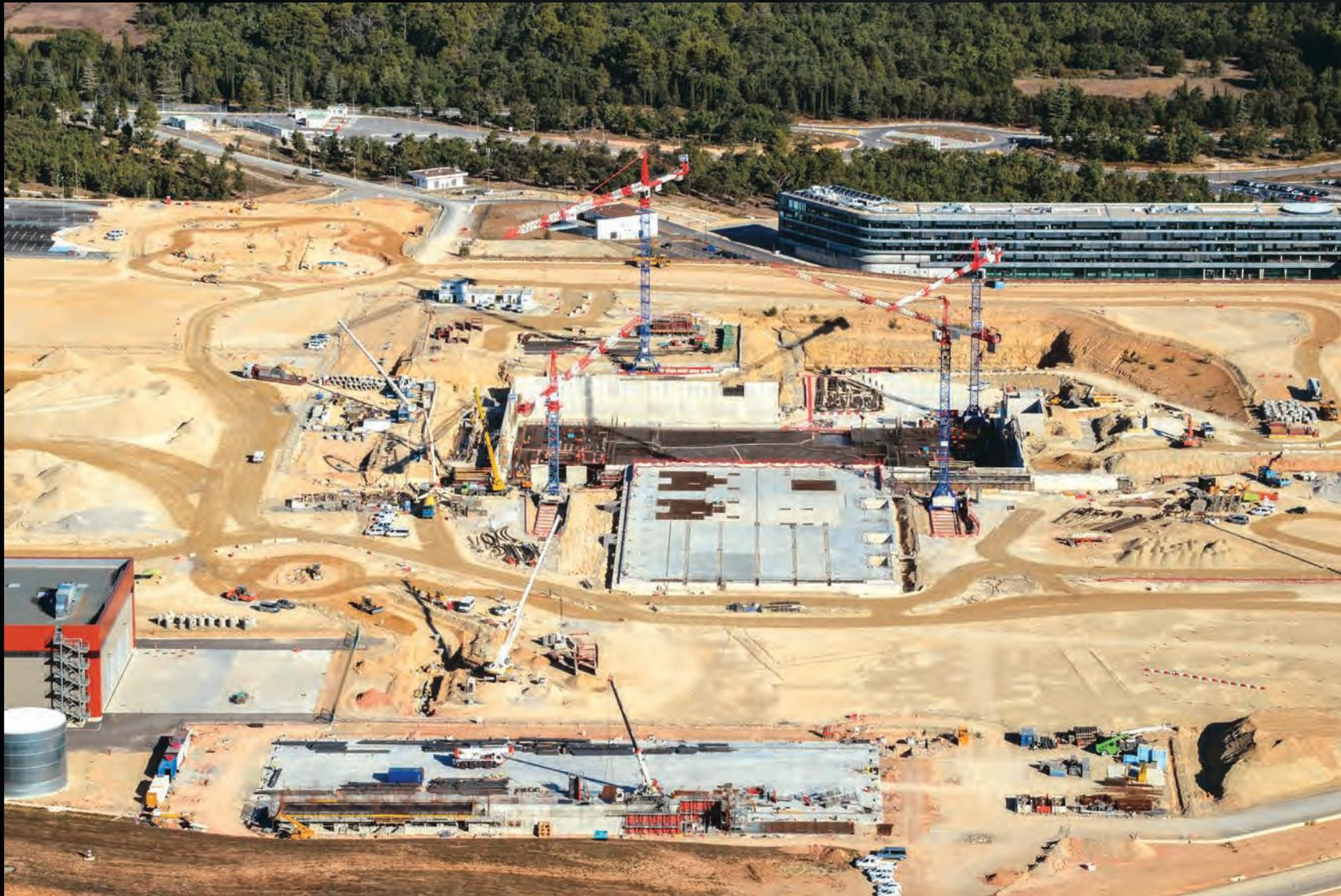
A partial view of the ITER platform in September 2013. The Poloidal Field Coils Winding Facility (bottom left) has been finalized; work is progressing on the Cryostat Workshop (foreground) and the Assembly Hall/Tokamak Complex (centre). Slightly below the level of the platform, ITER Headquarters, in the background, has office space for approximately 500 staff and contractors.
