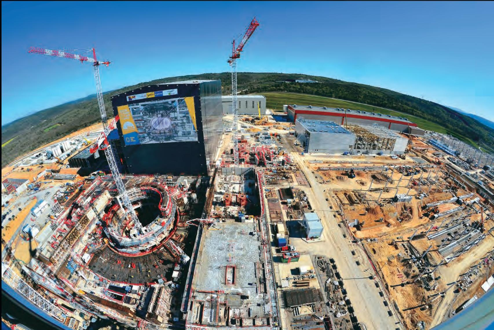
The ITER construction platform, seen from a worksite crane. The Assembly Hall is the most prominent feature, with the Tokamak Complex under construction right in front of it. Plant systems will be housed in buildings under construction across the rest of the platform. The poster on the Assembly Hall shows a cutaway of the ITER tokamak at 70% of its actual size.
