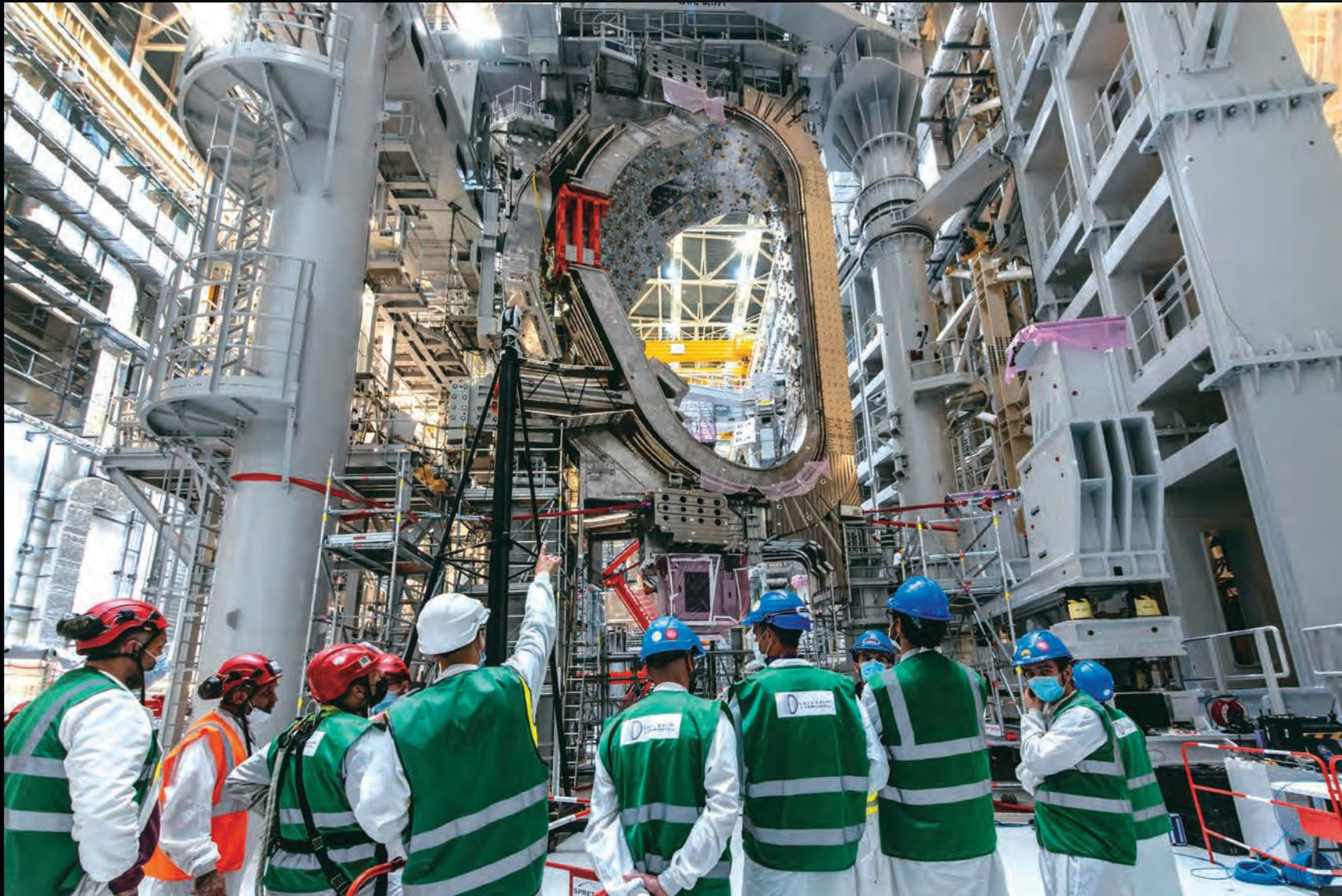
Vacuum vessel sector #6 is raised 50 centimetres and then redocked as part of a rehearsal for the big lift to come, which will bring the sector into the tokamak pit. The operation allows the teams to test rigging, sequences, and coordination.
