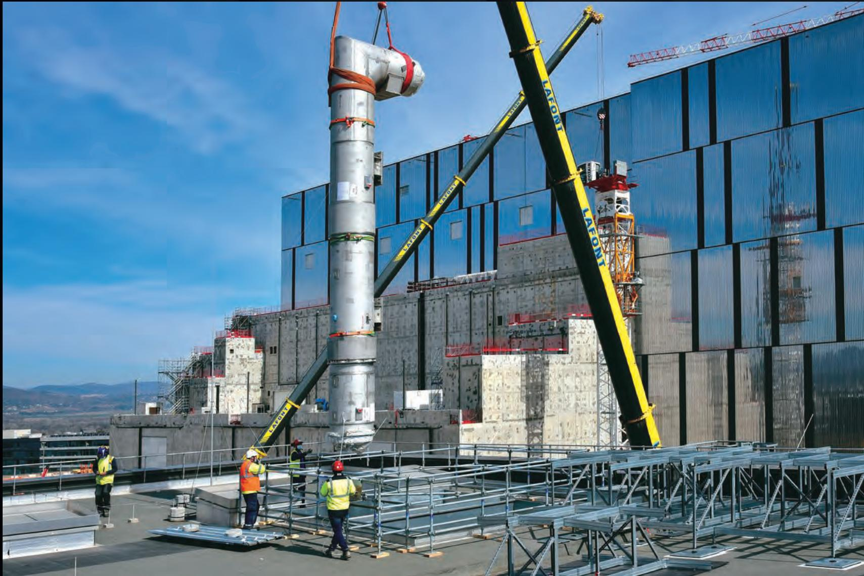
A cryoline spool is lowered into the ITER cryoplat, part of the multi-process piping system that will transport cooling fluids to the Tokamak Building in the background.
