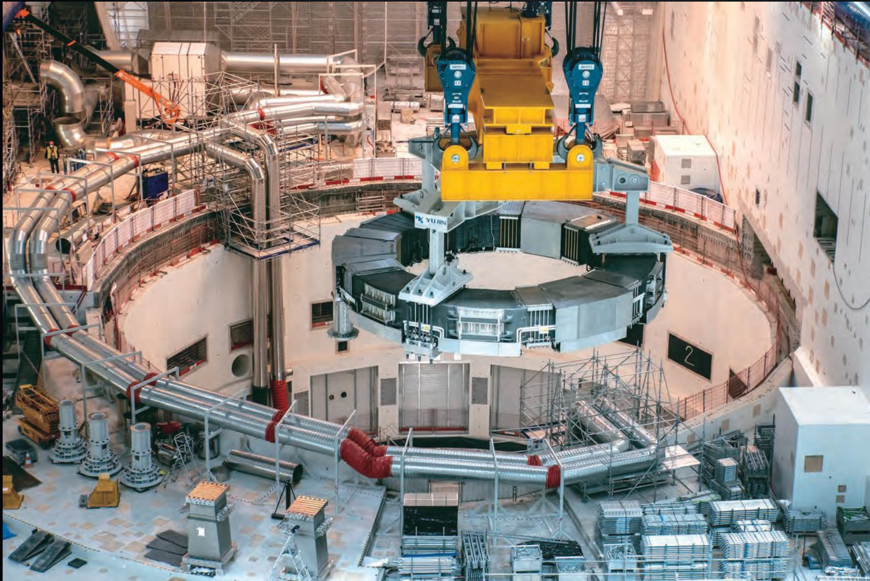
The installation of the first magnet, 330-tonne poloidal field coil PF6, is a major assembly milestone achieved in April.
