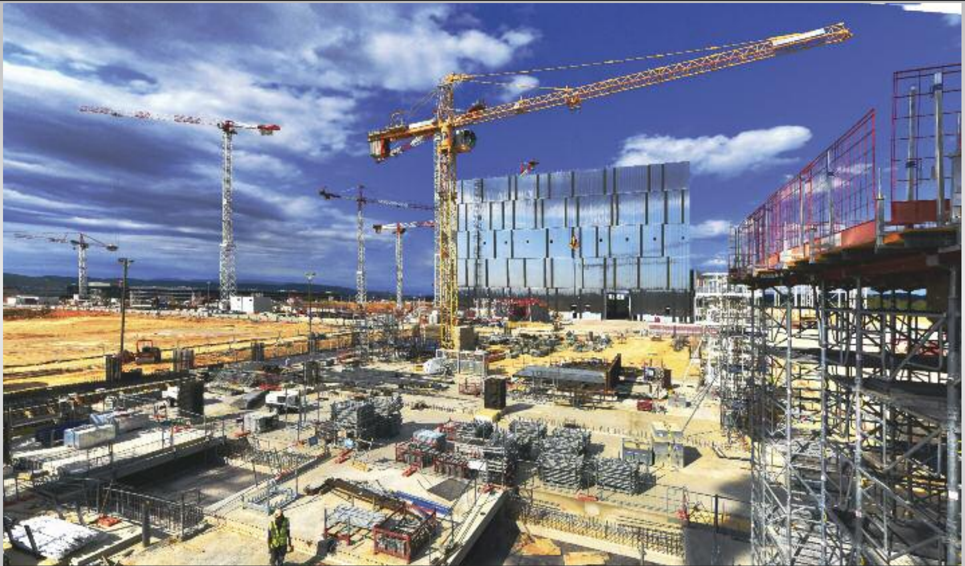
The ITER Cryoplant Building is under construction now on the southeast portion of the platform. In parallel, cryogenic components (cold boxes, turbines, compressors ...) have begun arriving on site. July 2016
