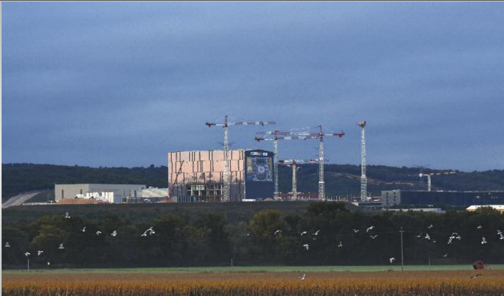
The Assembly Building will be equipped with specialized tooling to handle and pre-assemble Tokamak components. The building's mirror-like cladding, completed in 2016, will be reproduced on all the main buildings of the ITER facility. October 2016
