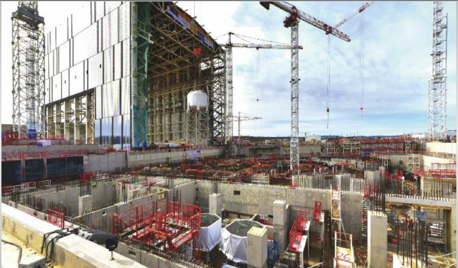
This water detritiation tank being lowered into the Tritium Building is one of six that have since been installed at the B2 (lower basement) level.
