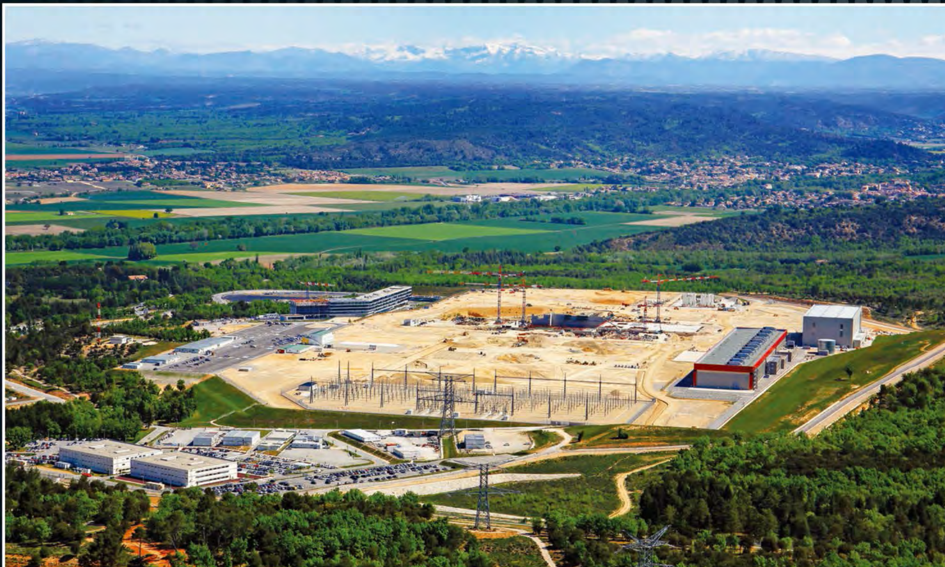
Looking north over the ITER worksite. April 2014
