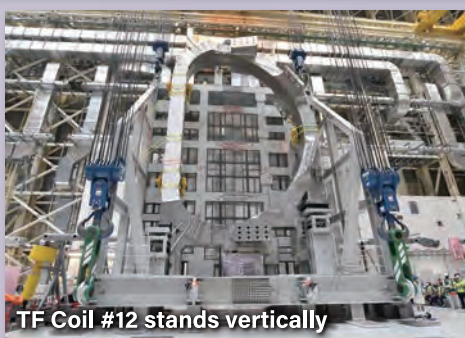
Installation of first sector sub-assembly
