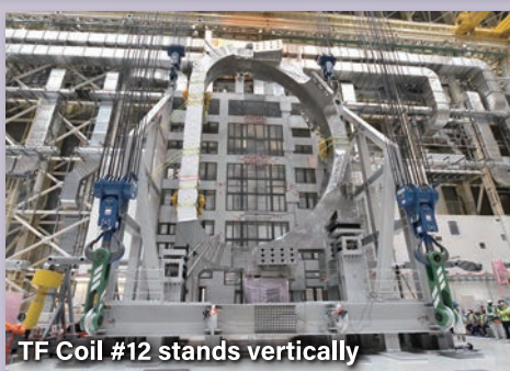
Installation of first sector sub-assembly
