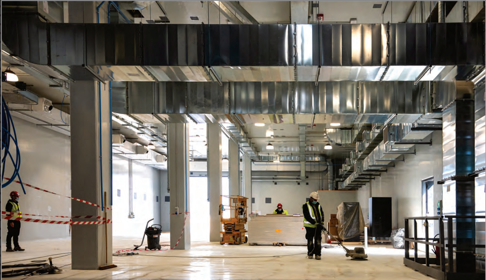
The Tokamak Assembly Preparation Building – designed for the storage and handling of ITER's beryllium components – is completed to nuclear standards in just nine months. The building will be used for pre-assembly activities until the blanket first-wall panels begin arriving in late 2024. December 2020
