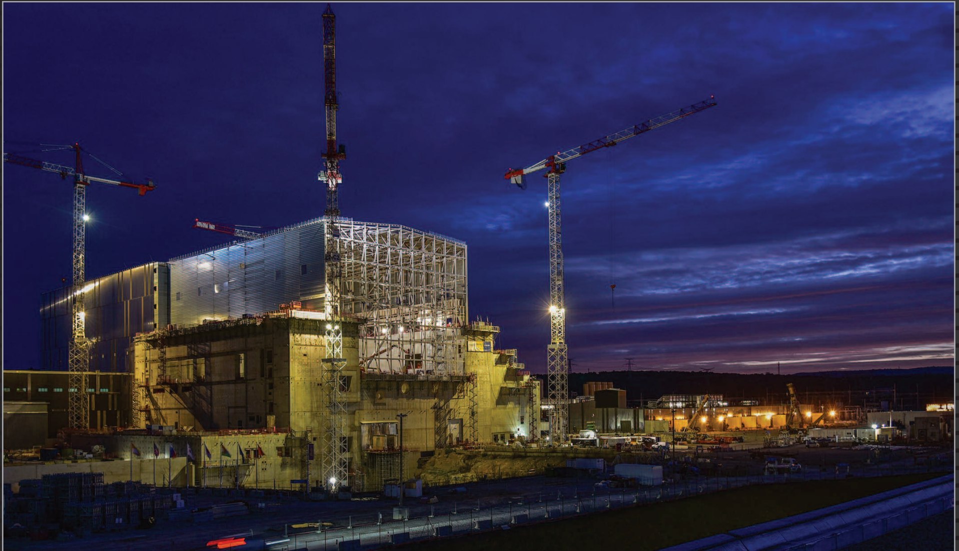
The European Domestic Agency completes the structure and cladding of the Tokamak Building crane hall early in the year, opening the way for machine assembly to begin. February 2020
