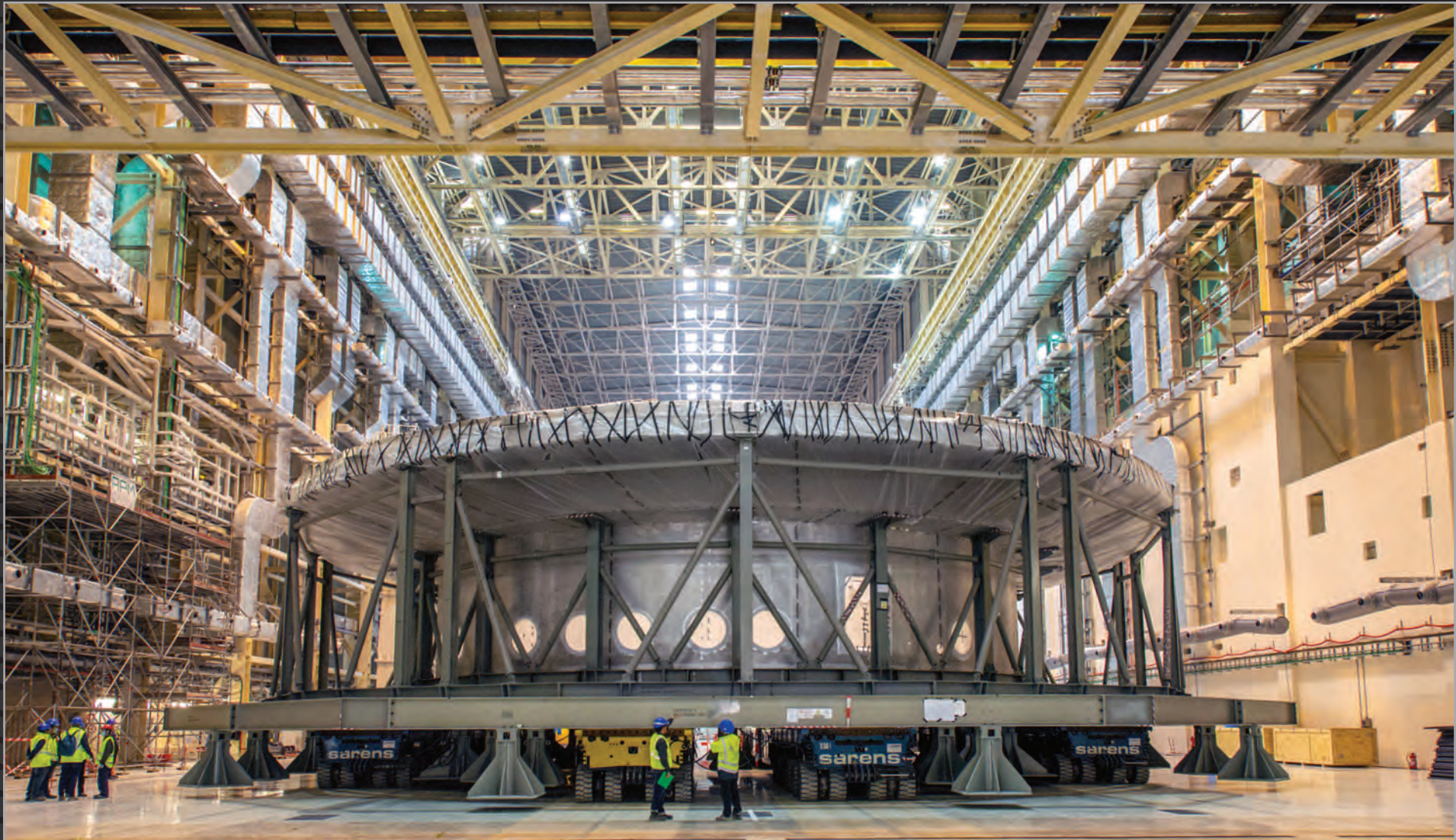
Months of careful preparation by metrology experts, cryostat engineers, crane operators, operational specialists, and supervisors are rewarded as the lift, transfer and insertion of the cryostat base goes off without a hitch. May 2020
