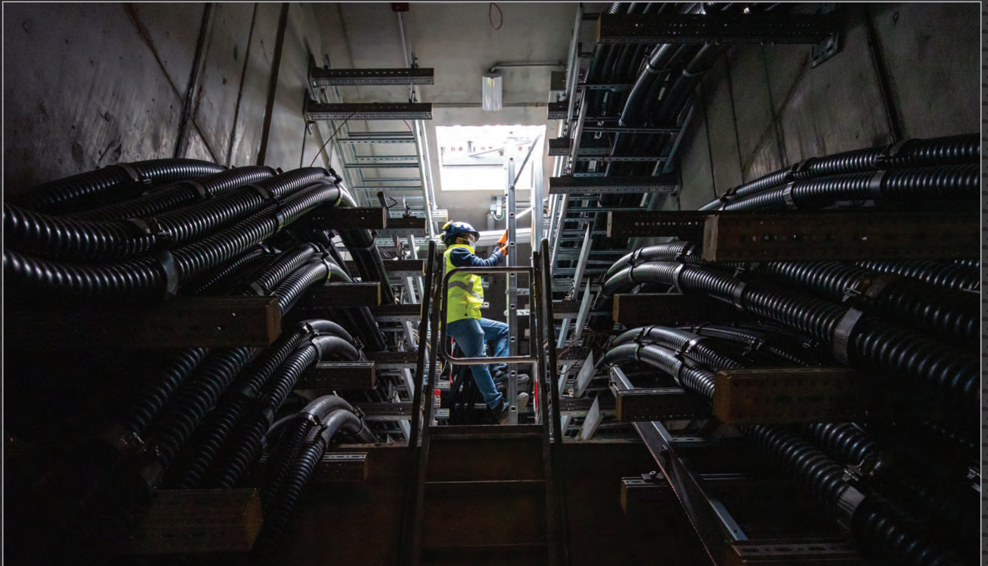
More than 4.5 kilometres of cable galleries run underneath the ITER construction site. In certain places, where the cables bend towards the surface, the impression is that of tentacles belonging to a creature lurking in the depths. December 2020
