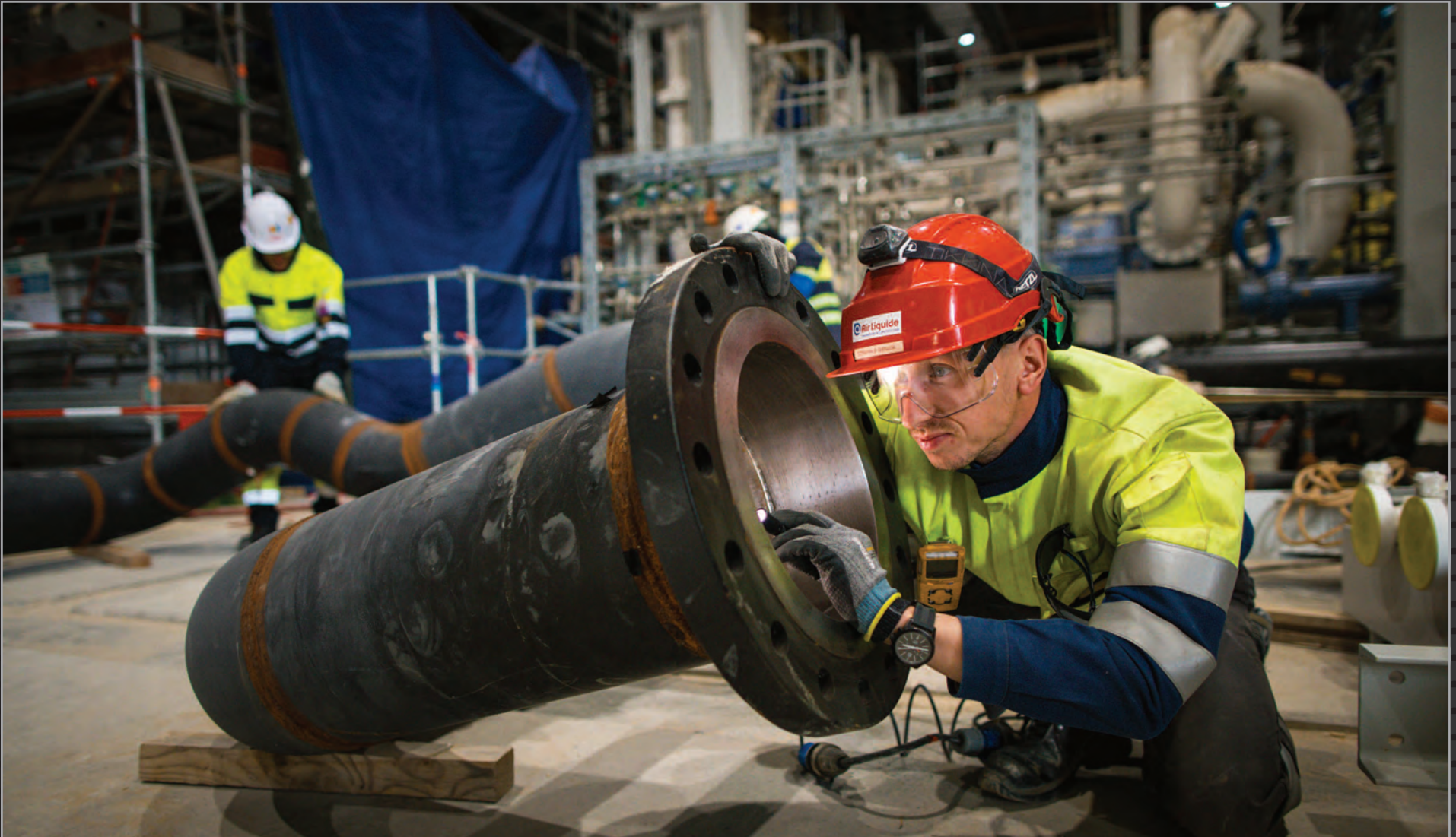
Europe has nearly completed the welding work for liquid nitrogen equipment in the cryoplant. Here, a pipe is inspected prior to installation.
