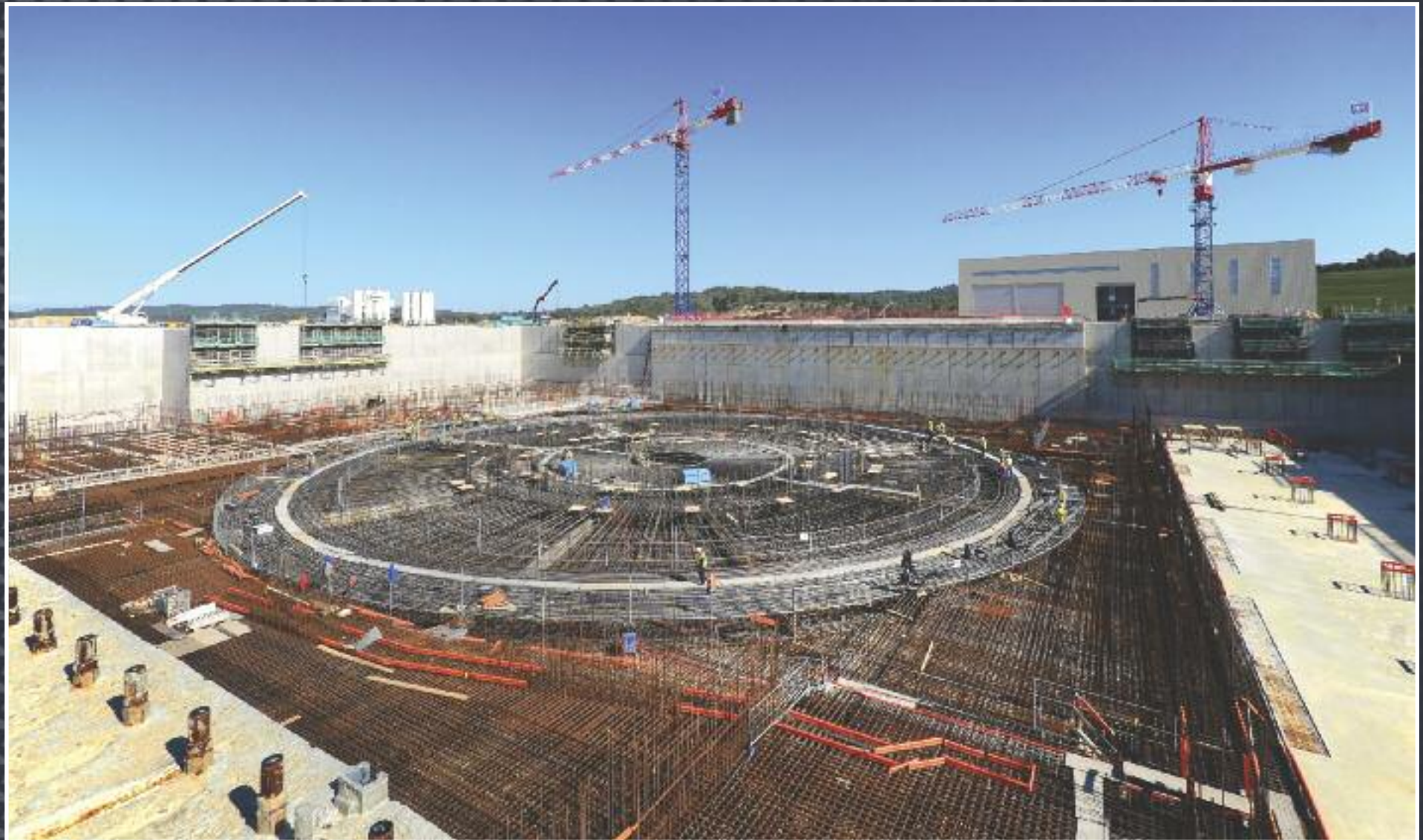
Rebar patterns are at their most complex in the centre of the Seismic Pit, where they will be part of the basemat supporting the ITER Tokamak. There, orthoradial (circular) and orthogonal (right-angled) rebar arrangements interface. April 2014
