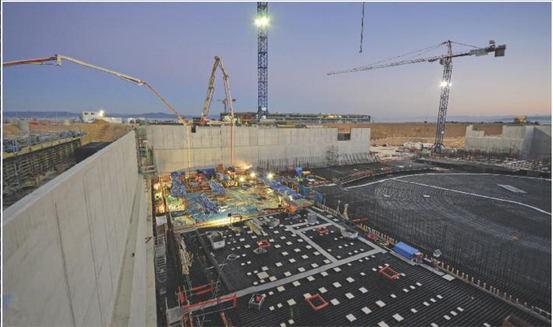
The Diagnostics Building will be situated at one end of the Seismic Pit. Work begins to pour the first of three basemat segments before dawn on 11 December 2013; the Diagnostics Building slab is completed in February 2014.
