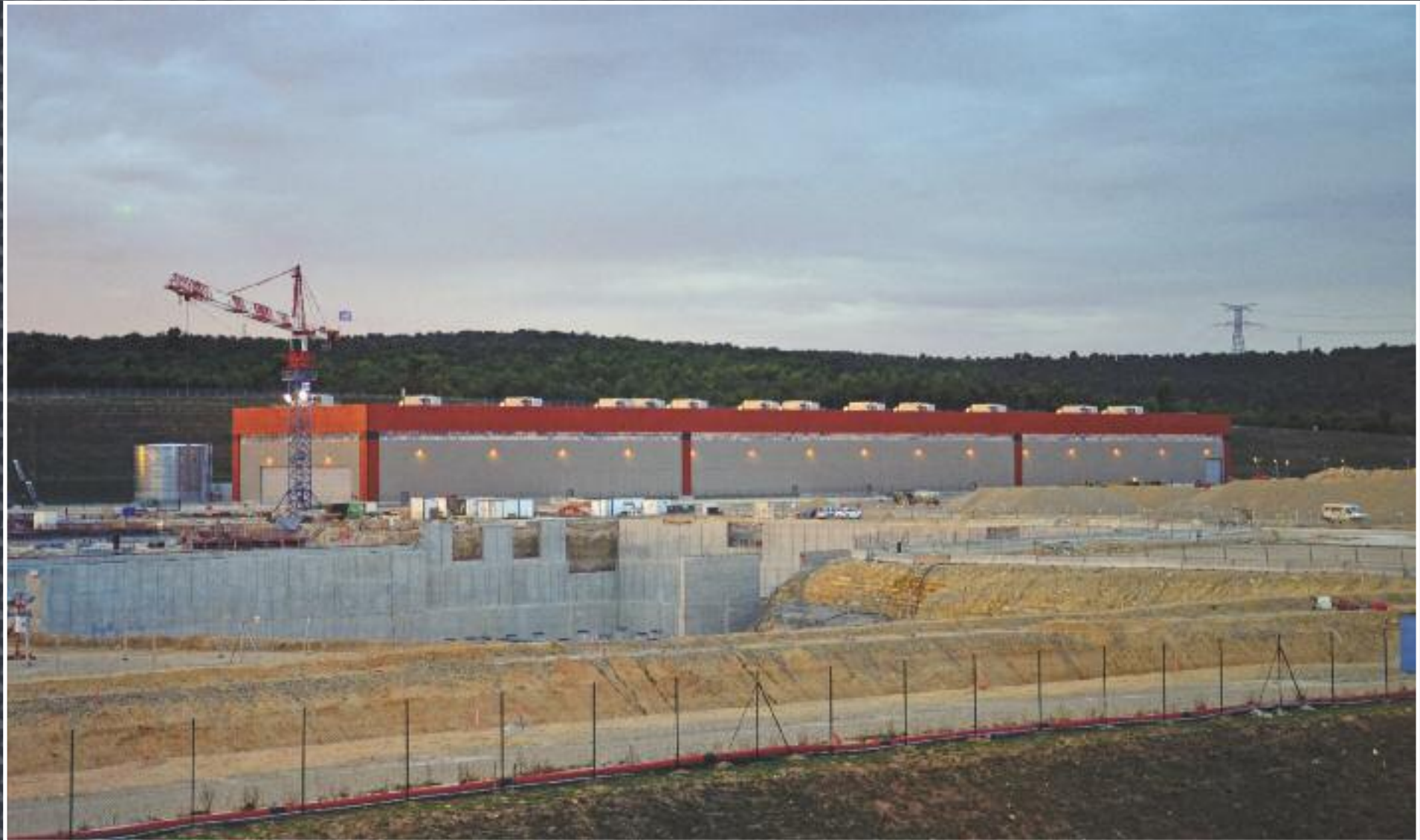
Too large to travel by road, four out of the Tokamak's six ring-shaped magnets (poloidal field coils) will be manufactured by Europe on site in this 257-metre-long, 49-metre-wide building. October 2012
