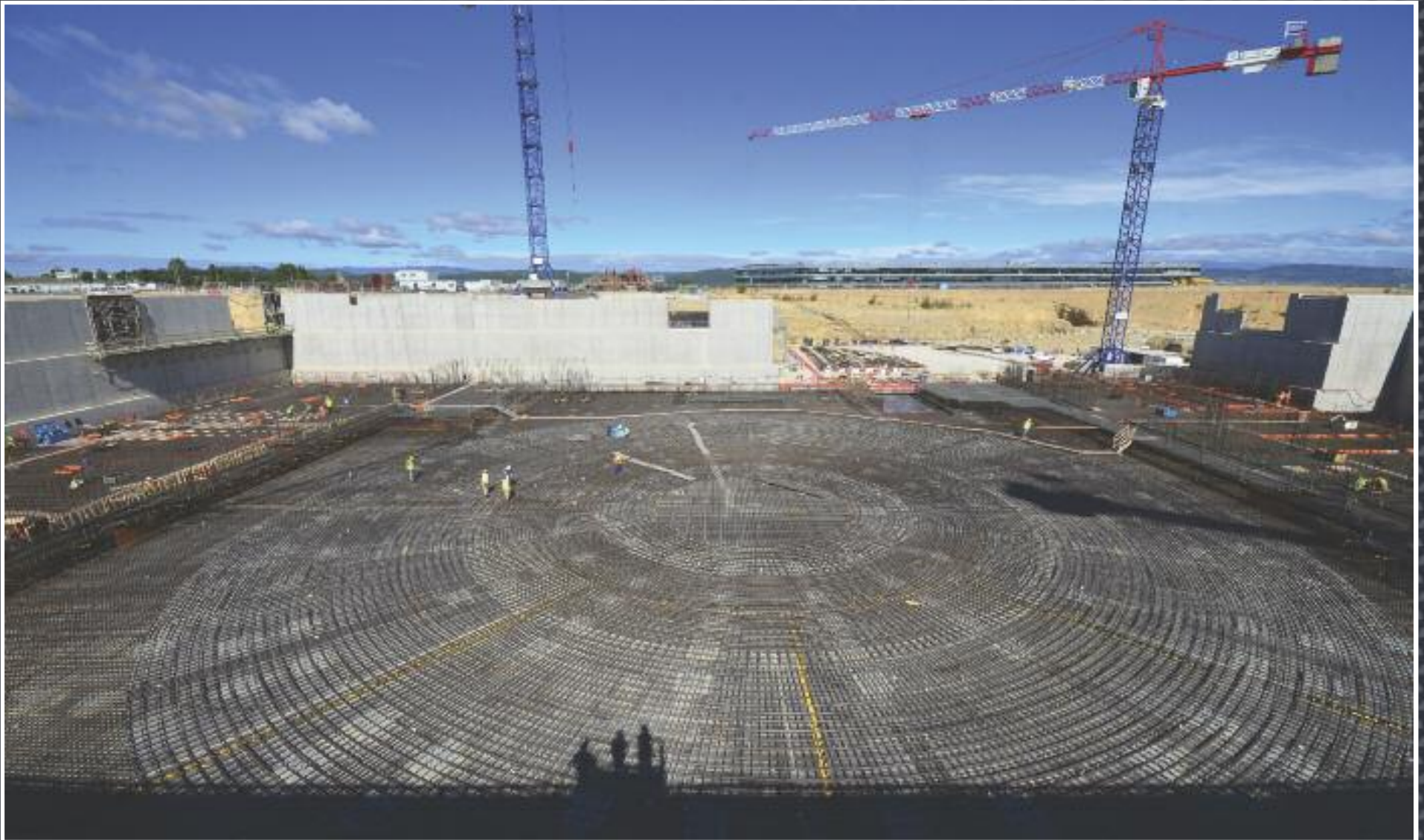
The antiseismic columns and pads are hidden from view by the formwork and reinforcement underway for the next-level basemat. The B2 slab will support the 400,000-ton Tokamak Complex. September 2013
