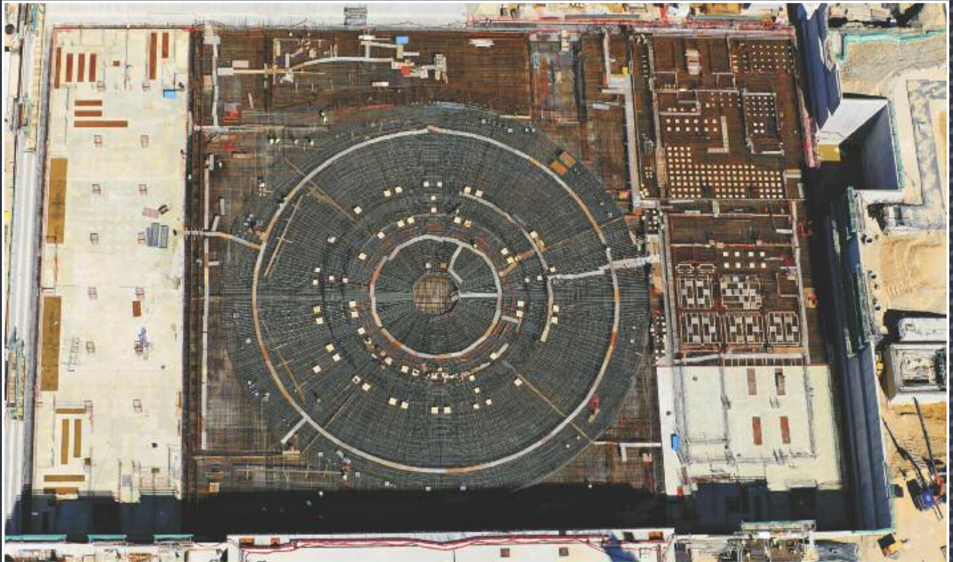
The Tokamak Complex is a suite of three buildings on a common foundation. On the left, the finished basemat slab of the Diagnostics Building. On the right, pouring is underway on the Tritium Building slab. In the central area, the circular pattern of rebar that will support the machine. April 2014
