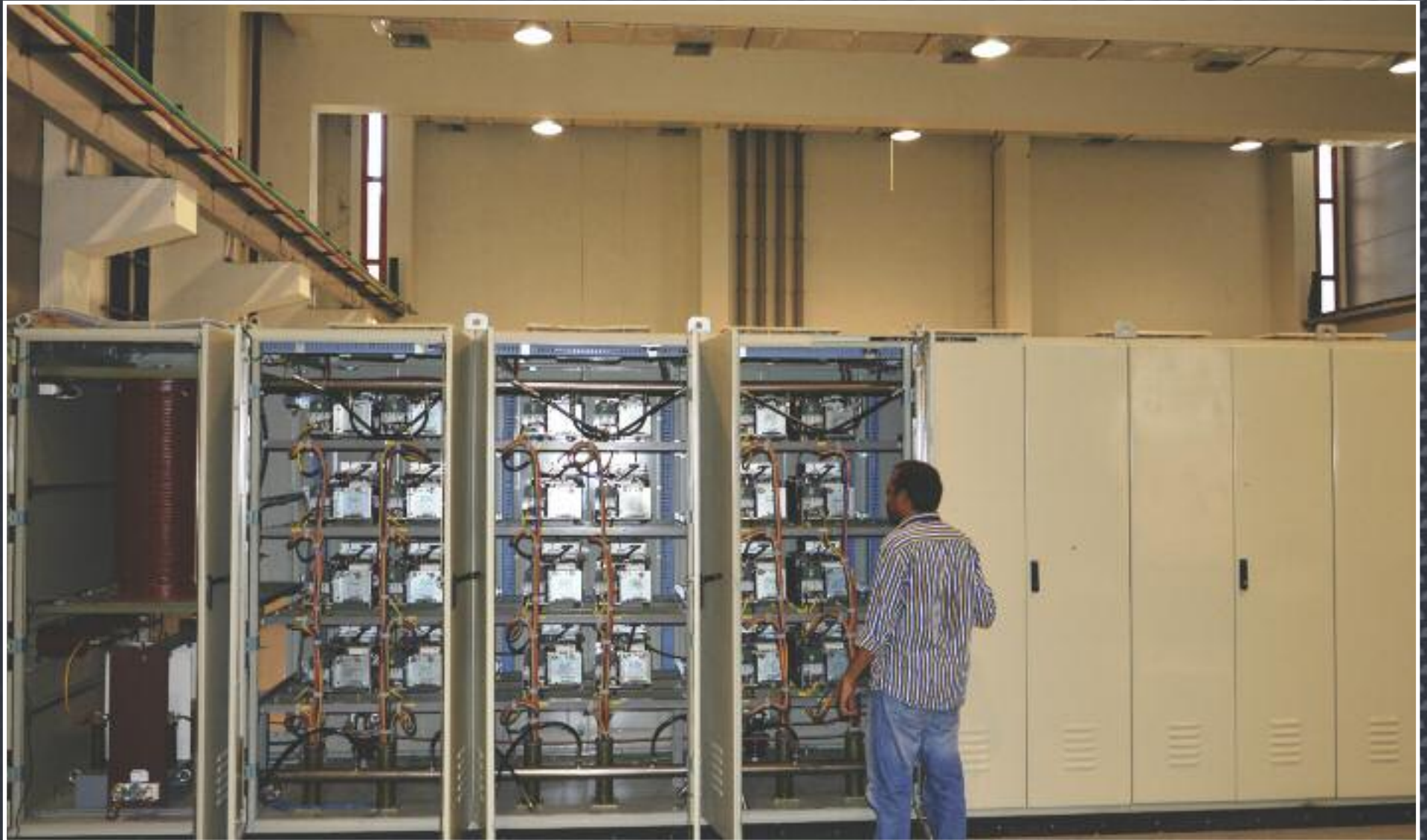
At ITER India, the high voltage power supply for ion cyclotron radio frequency heating (ICRH) is readied for testing.
