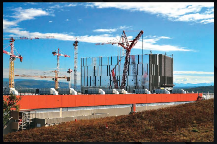
A massive crawler crane with a lifting capacity of 1,000 tonnes raises the steel girders of the Assembly Hall travelling cranes into position by passing hooks and cables through an opening in the roof.
