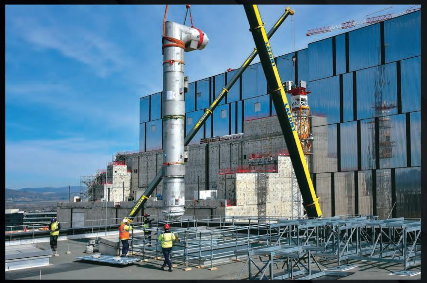
A cryoline spool is lowered into the ITER cryoplant, part of the multi-process piping system that will transport cooling fluids to the Tokamak Building in the background.
