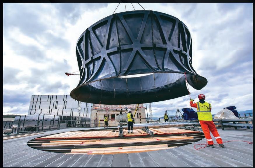
Each of the heat rejection system's 10 cooling cells is topped by a "fan cylinder" hosting a twelve-blade fan that will draw air upward and accelerate the evaporative process used to cool the water arriving from the installation's cooling loops.
