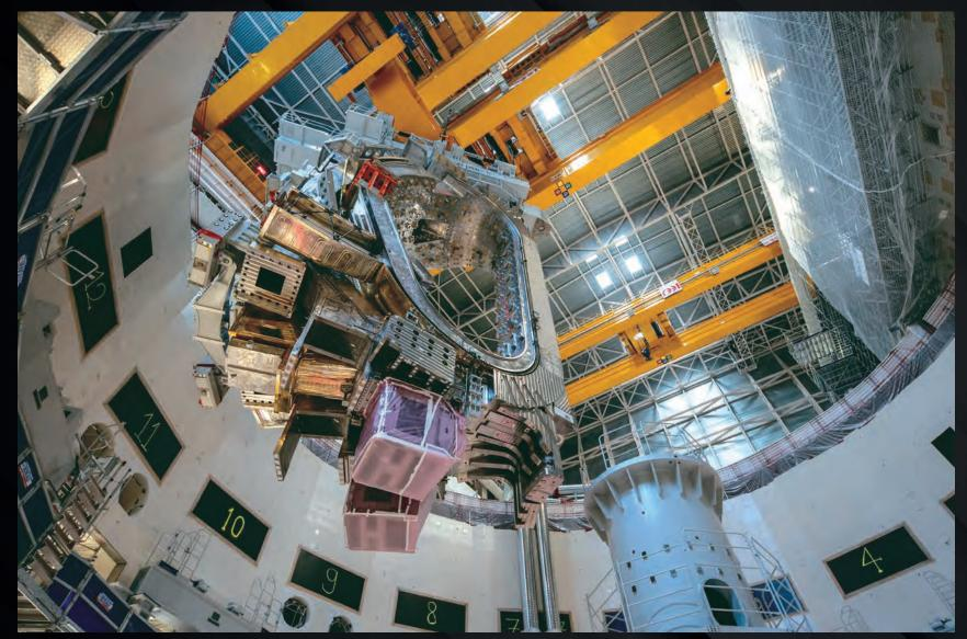
From detaching the module from its moorings in the assembly pit to lifting and transporting it to the sub-assembly tool, more than one hundred different steps were defined, validated and integrated into the lift procedure.
