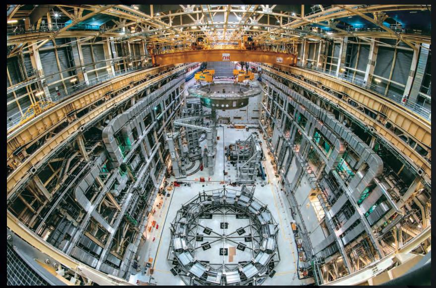
Ten years after building begins on the ITER site, the first machine component is installed in the tokamak pit in May-the 1,250-tonne cryostat base.
