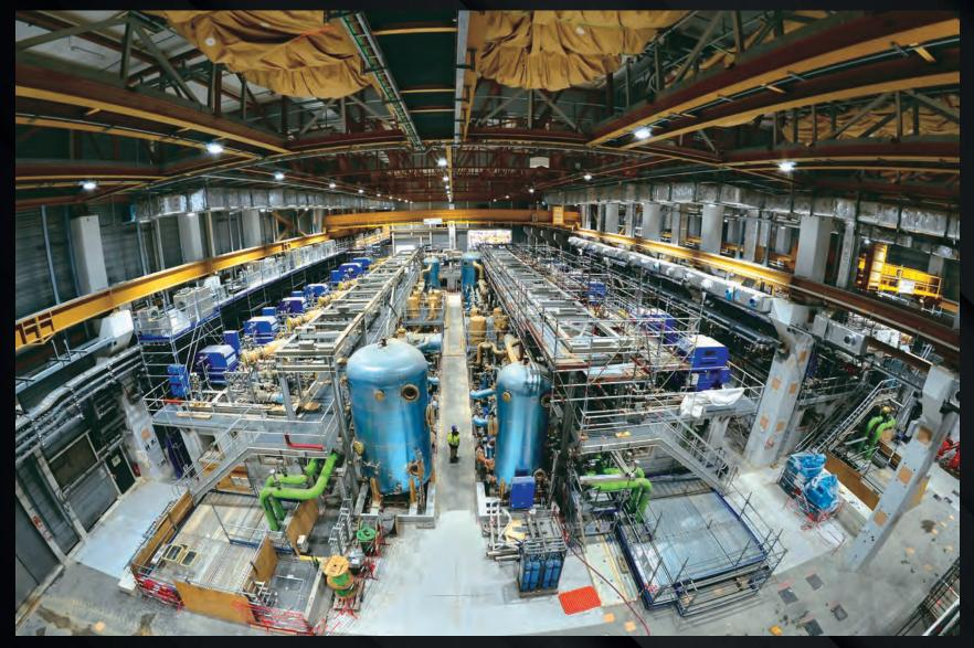
As large as two football pitches, the ITER cryoplant will provide cooling fluids to 10,000 tonnes of superconducting magnets, eight massive cryopumps, and thousands of square metres of thermal shielding.
