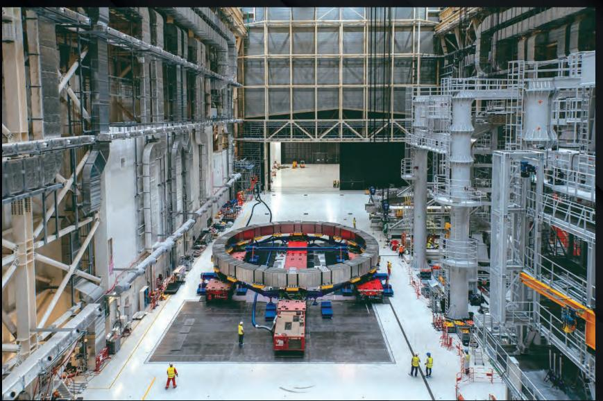
The double doors are closing behind poloidal field coil PF5, which has just been delivered from temporary storage into the Assembly Hall. It will be lifted from its modular transport vehicle and set on temporary supports until its installation in the tokamak pit.
