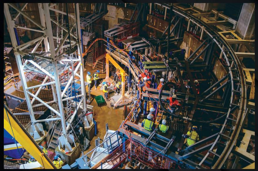
It is close to midnight in the basement of the ITER Tokamak Building and the first plot of the tokamak "crown" is to be poured. The operation is of strategic importance: the crown will support the combined mass of the tokamak and its encasing cryostat (23,000 tonnes) while transferring the forces and stresses generated during plasma operation to the ground.
