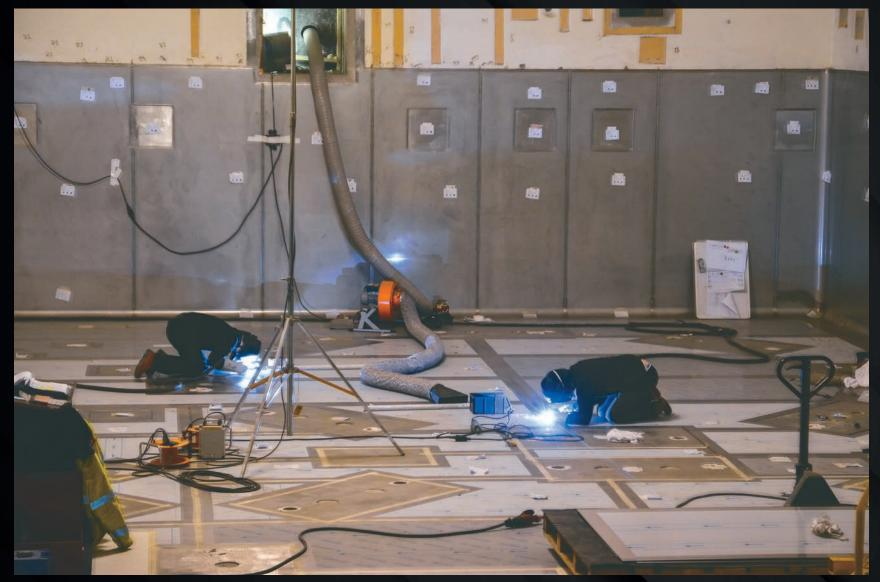
Deep in the bowels of the Tokamak Building, workers are busy lining the floor and the lower walls of the drain tank room with stainless steel panels. In case of a leak in the tokamak cooling water system, the lining will act as a "drip pan" to contain contaminated effluents.
