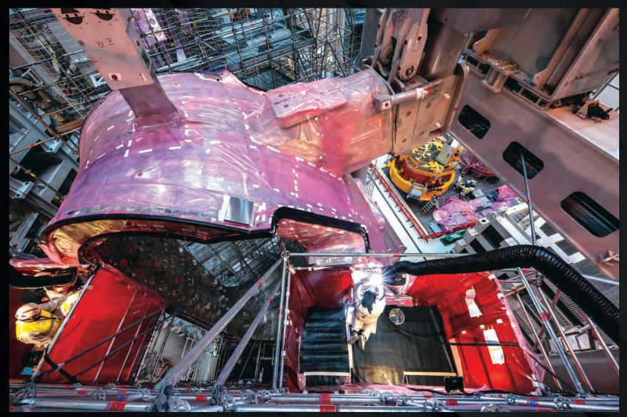
A campaign is underway to repair the dimensional non-conformities in the outer shell field joints of three vacuum vessel sectors. Pictured, scaffolding surrounds sector #7 as contractors work at four different levels to re-work the bevel joints by either building up missing material or shaving off excess material through machining.
