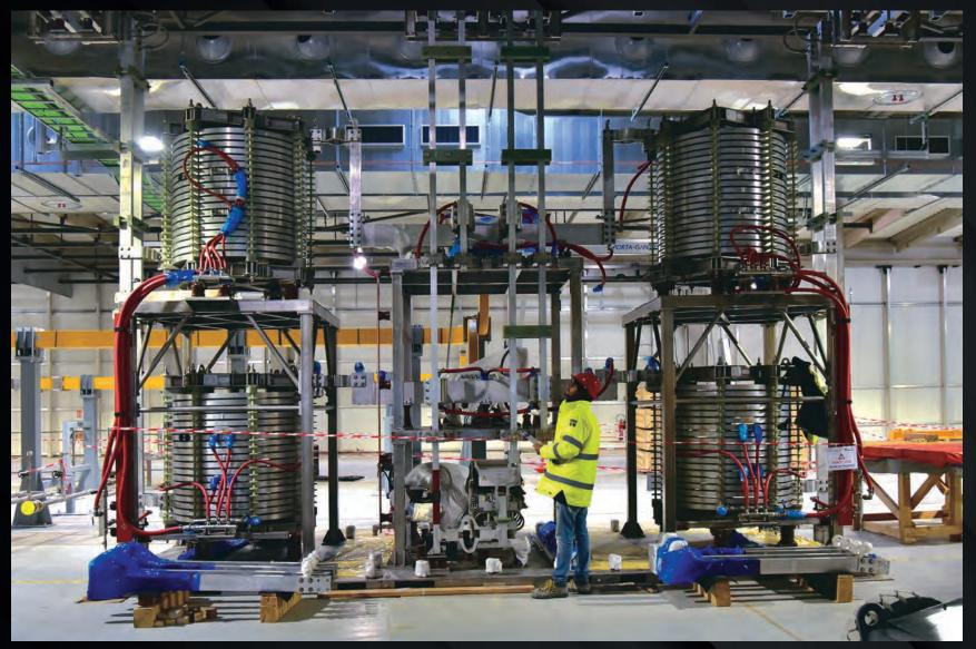
Twin buildings on site are filling up with equipment to convert AC power to DC power for the superconducting magnets. This strange contraption, a "reactor," creates a magnetic field to filter small spikes in DC waveform before it is fed to the magnetic system.
