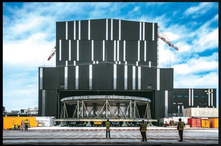
The doors of the Cleaning Facility open to admit the cryostat base in May. The assembly phase kicks off with the installation of this 1,250-tonne component, the heaviest of the ITER machine.
