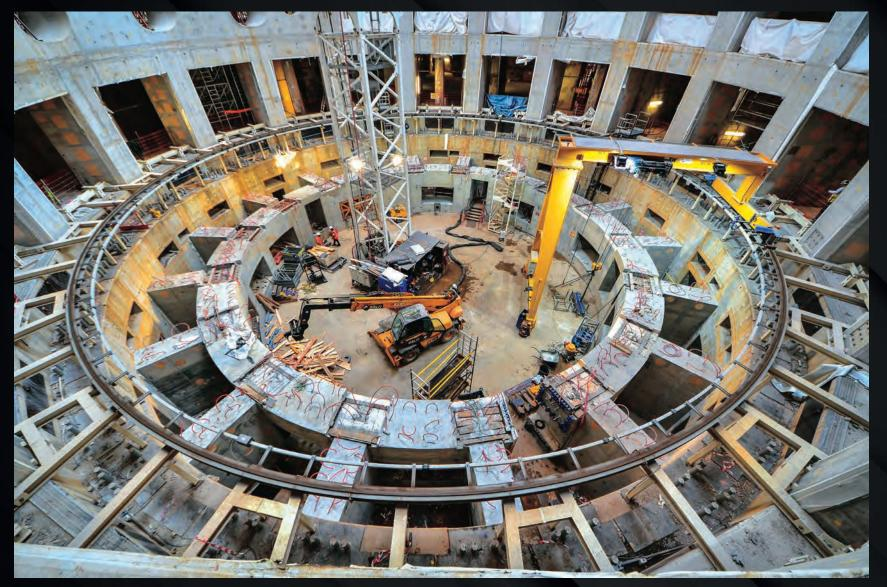
On the floor of the tokamak pit, European contractors prepare to pour the concrete crown - the ring wall foundation that will support the full weight of the machine.
