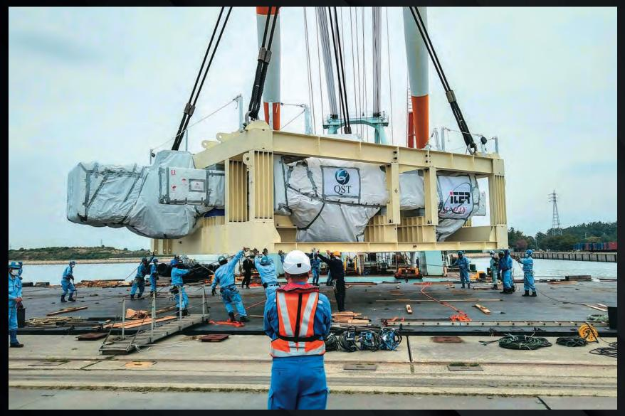
A toroidal field coil manufactured in Japan is prepped for loading at the Port of Kobe in April. Quality and safety must be strictly managed not only for coil fabrication but during transportation as well.
