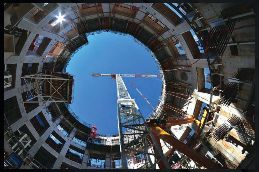
Inside the huge well of the ITER bioshield, construction teams are working on different levels simultaneously. Soon, a temporary steel cap—whose purpose is to protect teams below while allowing work to continue above—will split the volume in two.
