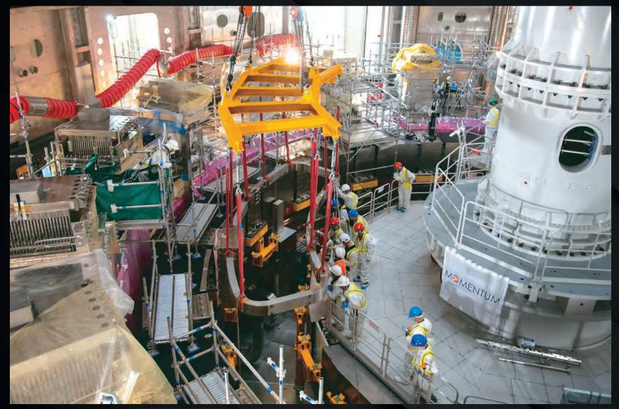
Eighteen small superconducting coils inserted between the major toroidal and poloidal field systems will help correct unwanted field perturbations that can affect plasma stability and confinement. All six bottom correction coils have been installed.
