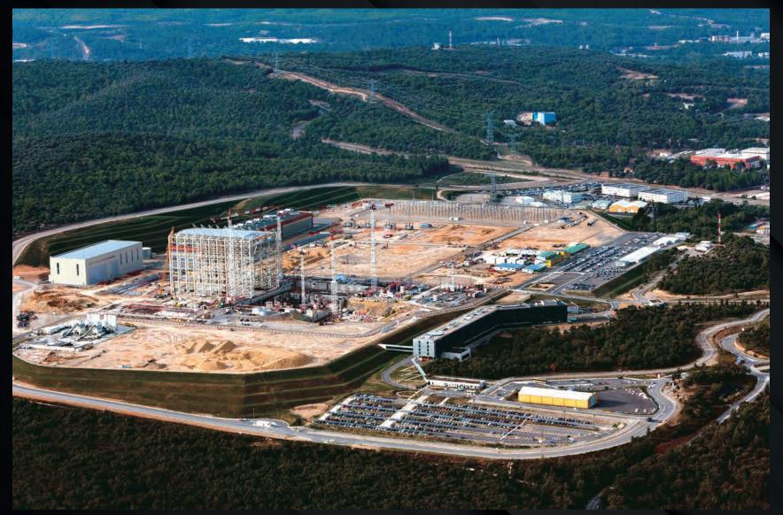
Since the completion of its metal structure the Assembly Building is the tallest building on the ITER platform, rising 60 metres above ground level. Here pre-assembly activities will be carried out on the principal tokamak components prior to installation.
