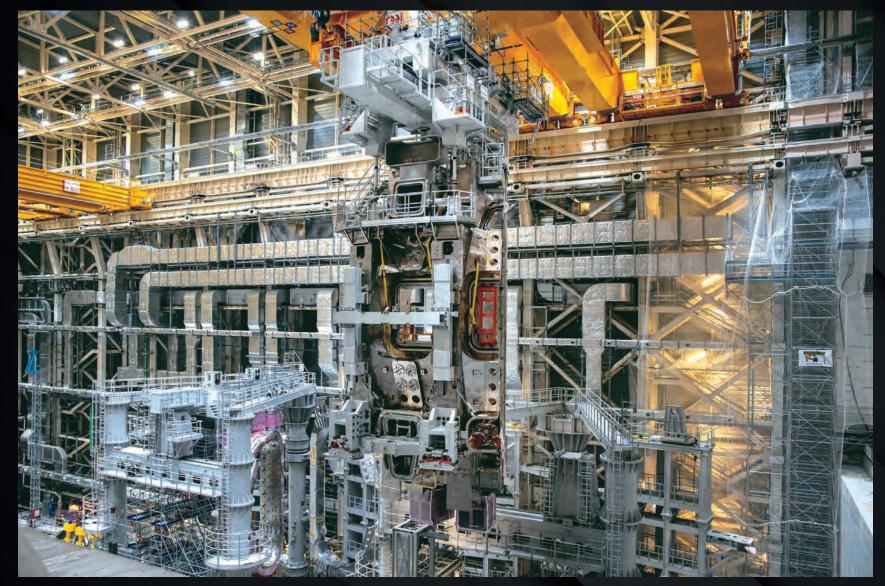
The first-completed sector module—sector #6, 1,380 tonnes—is lifted out of tooling in the Assembly Hall. It takes two days to extract the module, transport it over the wall to the tokamak pit, and position it with sub-millimetric precision on supports.
