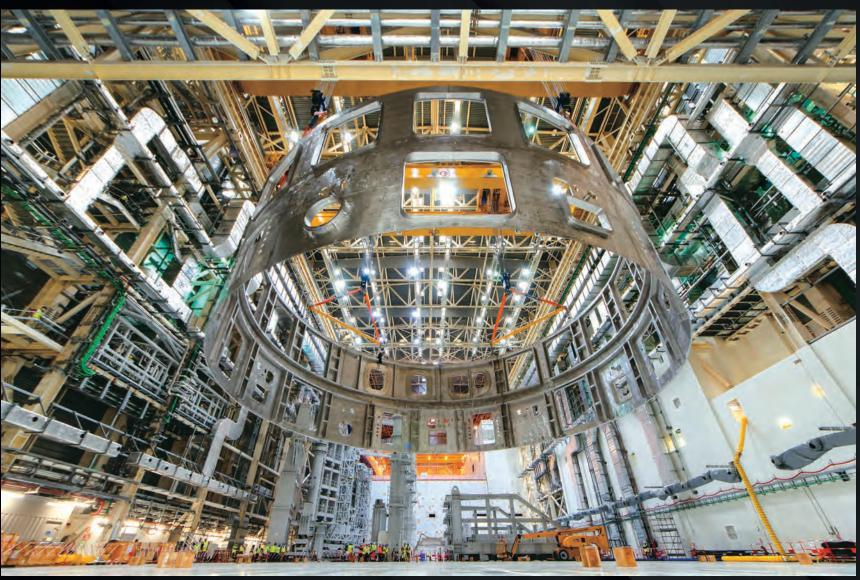
After the cryostat base in May, the cryostat lower cylinder is successfully installed in August. The steel ring, although much taller than the base (12 vs 4 metres), is a considerably lighter load at 375 tonnes (vs 1,250).
