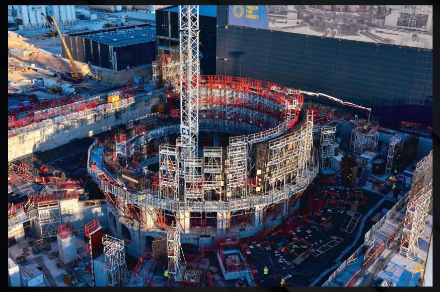
Concrete pouring is underway to complete the ITER bioshield before the first captive components are installed. The assembly of the world's largest tokamak will take place from bottom up – starting with the cryostat base and ending with the cryostat lid.
