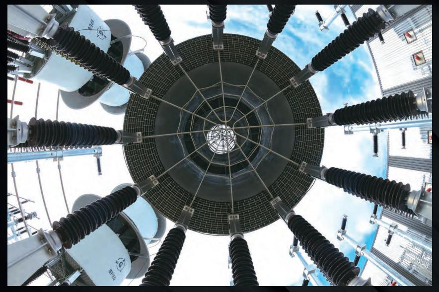
This alien-looking object is part of ITER's reactive power compensation and harmonic filtering system, designed to reduce "harmonic distortions" in the AC current that ITER receives from the grid.
