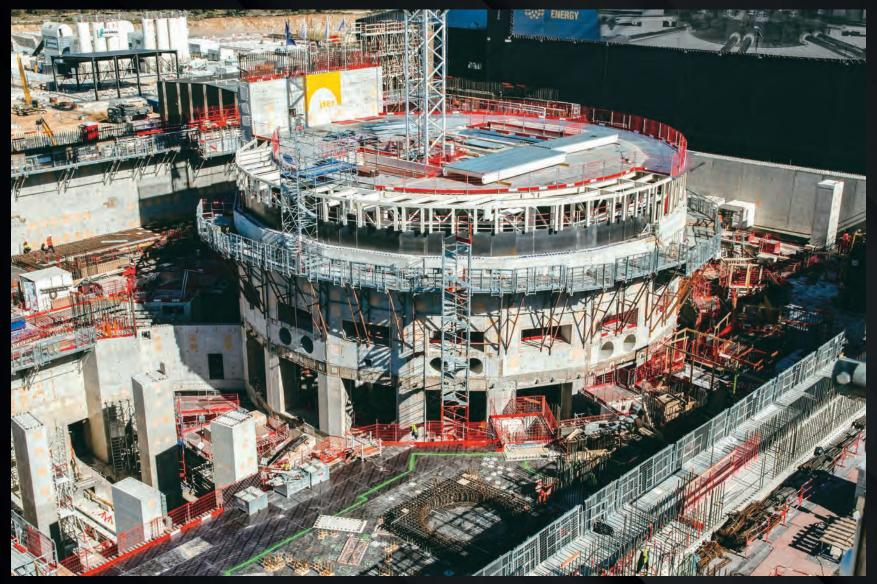
The lid is raised to the top of the bioshield in March, becoming a protective roof for all activities below. Teams can now work freely in the 30-metre-deep machine assembly arena.
