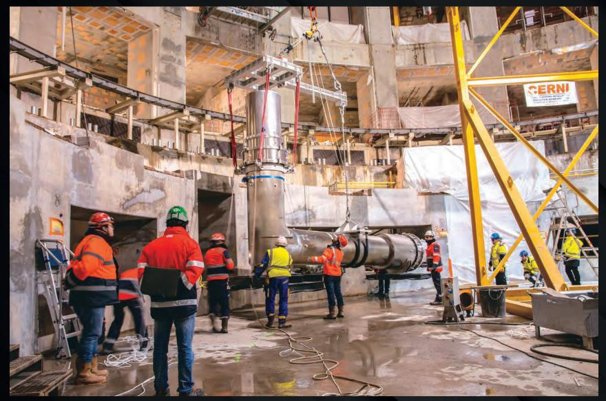
A 10-metre, 6.6-tonne magnet feeder segment from China is the first machine component to be installed in the tokamak pit.
