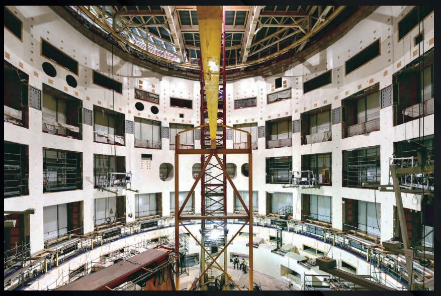
Raw concrete in the tokamak assembly pit has given way to the smooth shiny surface of many layers of white paint. The pit's vast volume (25,000 m<sup>3</sup>) is nearly ready to receive the first major machine components.
