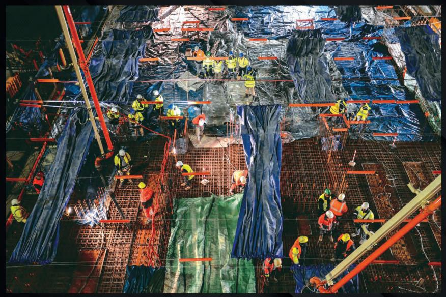
In December 2013, concrete pouring begins for the B2 basemat slab of the 400,000-tonne Tokamak Complex—a suite of buildings that includes the Tokamak Building, the Tritium Building and the Diagnostics Building.
