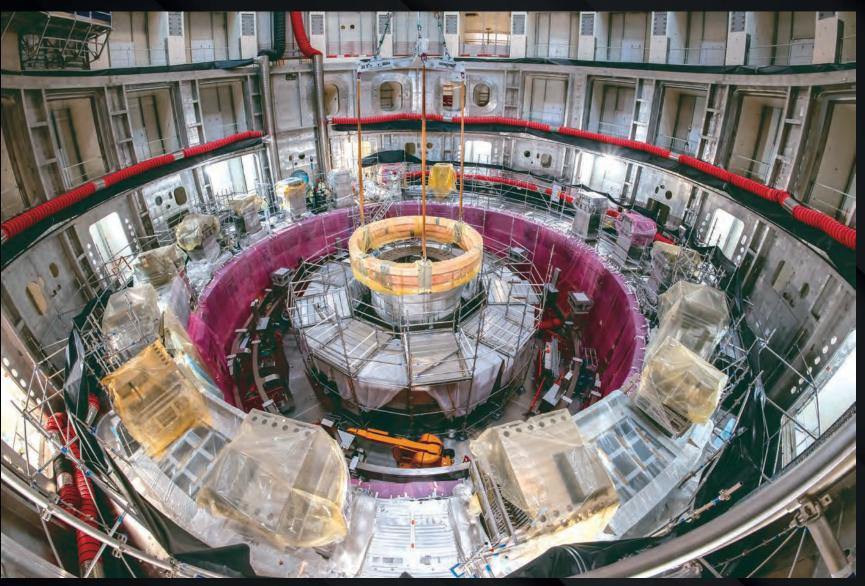
Procured by Europe, pre-compression rings like those in the centre of this image are part of the ITER magnet system. Made of glass fibre/epoxy composite, they will tightly hold the toroidal field coils at top and bottom with a radial force of 7,000 tonnes per coil. Two sets of three are required for operation; pictured is a spare set that was inserted at the bottom of the assembly pit in July.
