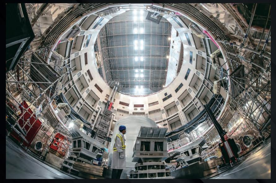
Core machine assembly started in May 2020. The cryostat base and lower cylinder, the lower cryostat thermal shield, and the gravity supports for toroidal field coils have been installed and temporary supports are ready to receive poloidal field coil PF6.
