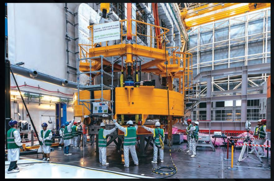
The central solenoid "stack" is taking shape in the Assembly Hall. In April, the third module is lifted with the aid of a bespoke lift tool and positioned over the two modules already in place. Six modules in all will create the 18-metre-tall central solenoid magnet.
