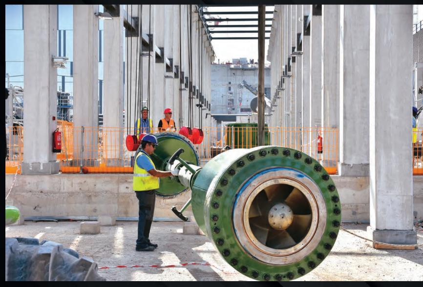
The amount of water that needs to be circulated within the heat rejection system is huge—in the range of 10 m<sup>3</sup> per second. Thirteen vertical turbine pumps, submerged deep in the basins, are tasked with moving one tonne of water per second per pump. Pictured: the installation of a 10-metre-long shaft for one of the turbines.
