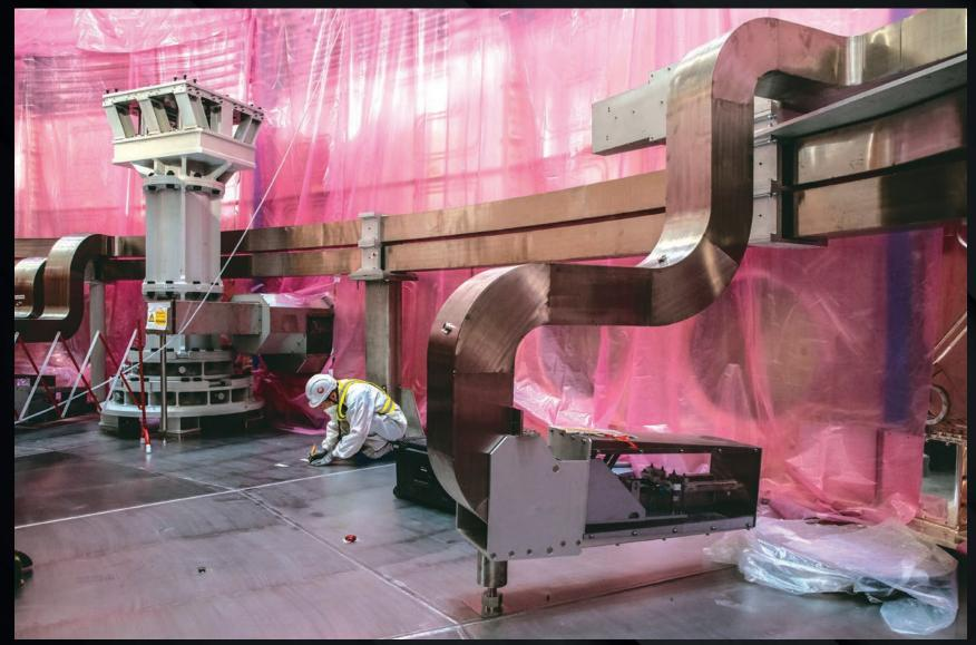
In 2021, the assembly pit is declared "ready" for the first vacuum vessel sector after all captive components (like the magnet feeders pictured here) are installed.
