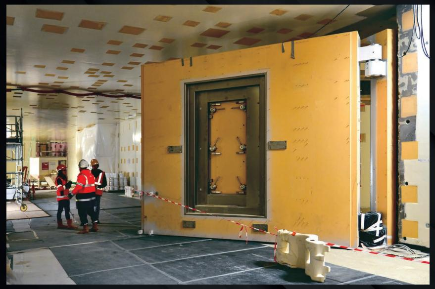
Forty-six port cell doors will seal off every port cell in the Tokamak Building, acting as confinement barriers to shield the environment from the radiation generated by the burning plasma. Each steel door is filled with 7.5 m<sup>3</sup> of high-density concrete.
