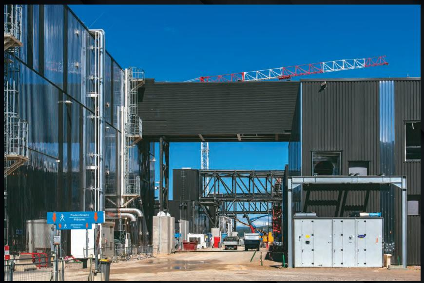
Cooling fluids and DC current leaving their production sites will be transported across elevated steel structures referred to as "bridges" to reach the Tokamak Building. Each one will support hundreds of tonnes of equipment.
