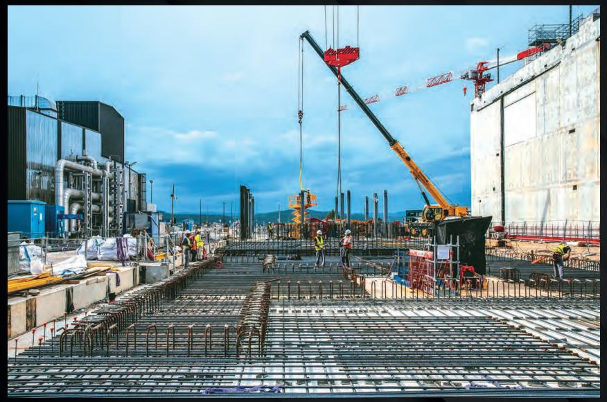
The bulk of infrastructure needed for the start of research operations is finished, but here and there on the worksite smaller buildings are still in construction. Pictured: teams work on the foundations of two electrical distribution buildings.
