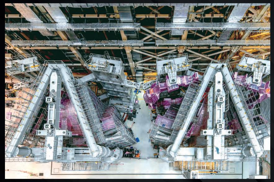
Seen from the Assembly Hall rafters: repairs are carried out simultaneously on vacuum vessel sectors #7 and #6. Work on sector #7 (left) is nearly completed, signifying that the sub-assembly process can be restarted soon.
