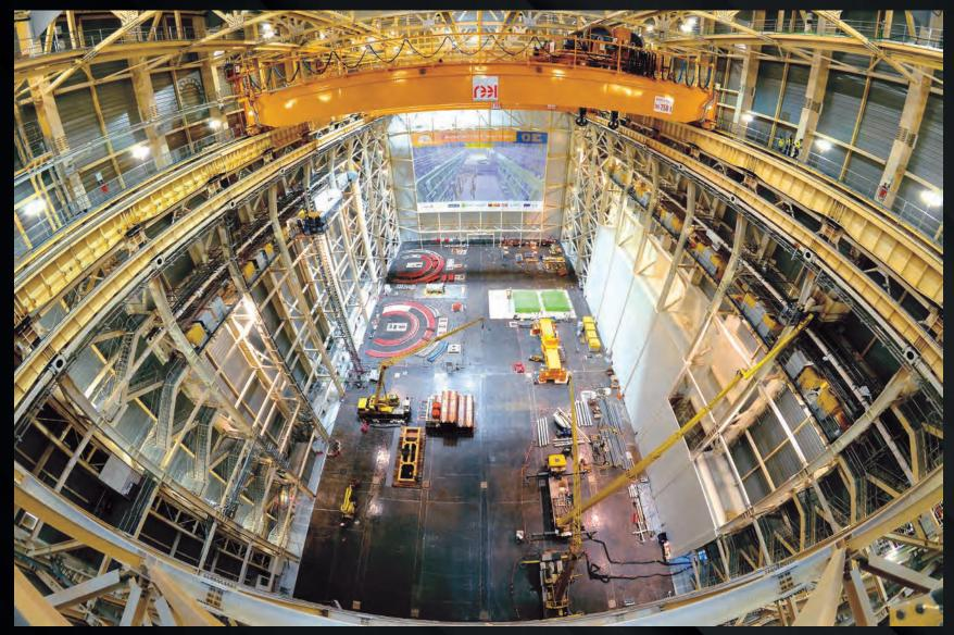
The ITER Assembly Hall is the space for the pre-assembly of all main machine components. As soon as the Tokamak Building is completed (far end) the temporary wall will be removed, giving direct access to the tokamak assembly pit.
