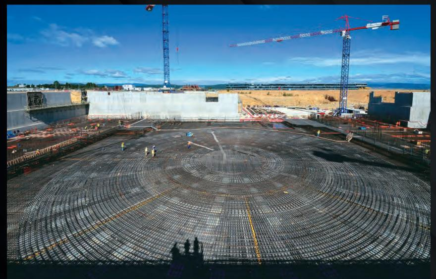
Contractors are preparing to pour 15,000 m<sup>3</sup> of concrete for the "floor" of the Tokamak Complex—the 1.5-metre-thick B2 slab. With rebar, the B2 slab weighs 37,500 tonnes, a load that is supported by 493 seismic pillars.
