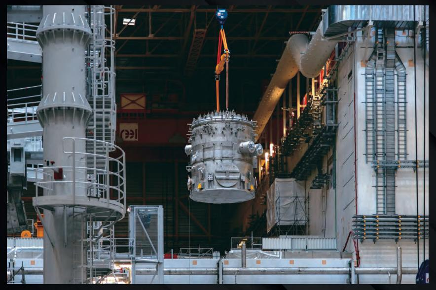
Installation activities are progressing full speed in the Tokamak Complex. Here, the first of the five auxiliary cold boxes required to distribute cooling fluids to different "clients" inside the machine is transferred into the Tokamak Building.
