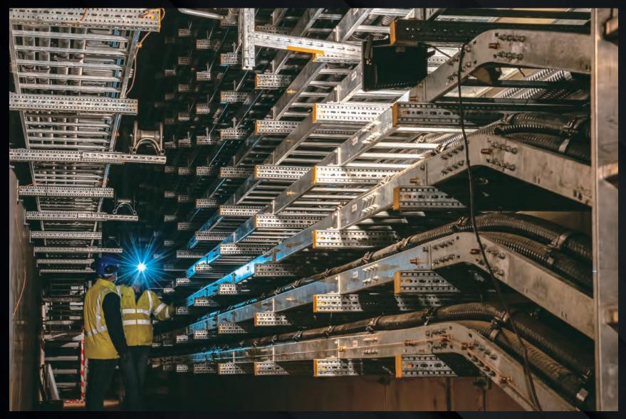
Put end to end, the electrical cables that crisscross the ITER scientific installation could reach the Peruvian capital Lima from the south of France—a total of 10,000 kilometres. Part of the 66kV underground network is shown here.
