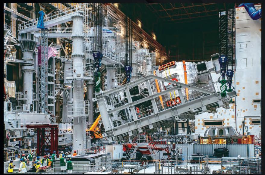
Some of ITER's most spectacular bespoke tools are in action in the Assembly Hall, where pre-assembly activities are carried out on the largest components of the ITER machine. In this photo, the "upending" tool transfers a 440-tonne vacuum sector from horizontal to vertical.
