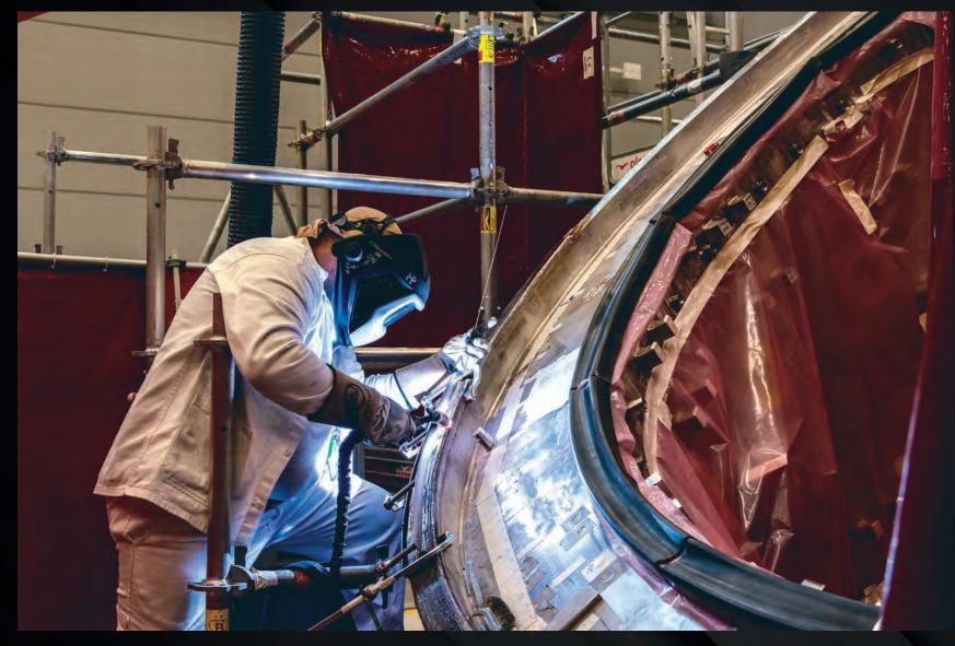
Vacuum vessel repair is being carried out at ITER by the SIMANN consortium (SIMIC S.p.A. and Ansaldo Nucleare). Repairs only began after the group had qualified its design solution and tools with mock-ups.
