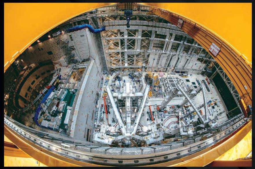
Taken from high above, this fisheye view shows the first vacuum vessel module, comprising components from Korea and Japan, being assembled in one of the twin sector sub-assembly tools.
