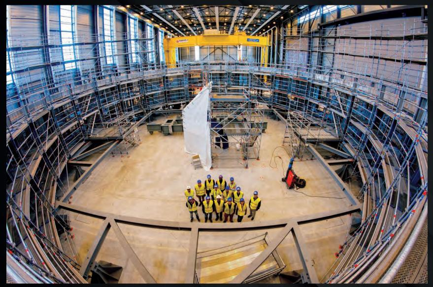
The ITER cryostat – the leak-tight vacuum container that will act as a thermos to insulate the ultra-cold superconducting magnets from the outside environment – is being assembled in a dedicated facility on site by contractors to the Indian Domestic Agency.
