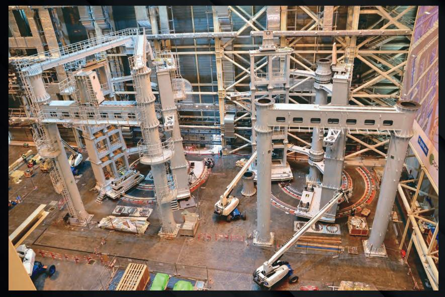
A second vacuum vessel sector handling tool has been delivered by Korea and installed in the Assembly Hall. The twin tools will be load-tested in early 2019.
