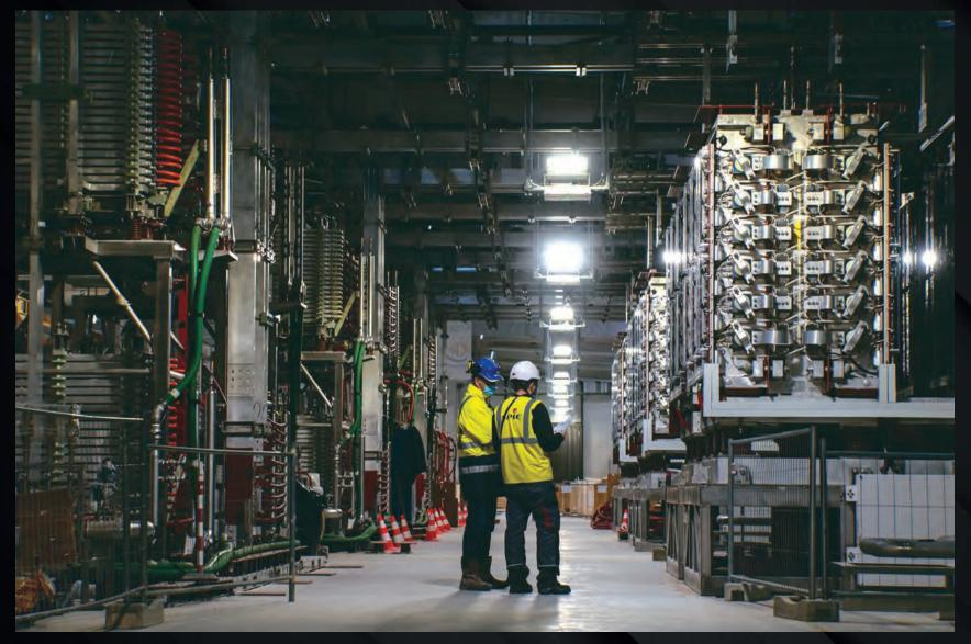
Twin buildings on site are filling up with equipment to convert AC power to DC power for the superconducting magnets. This converter from Korea will is part of equipment that will feed power to the vertical stability coils.
