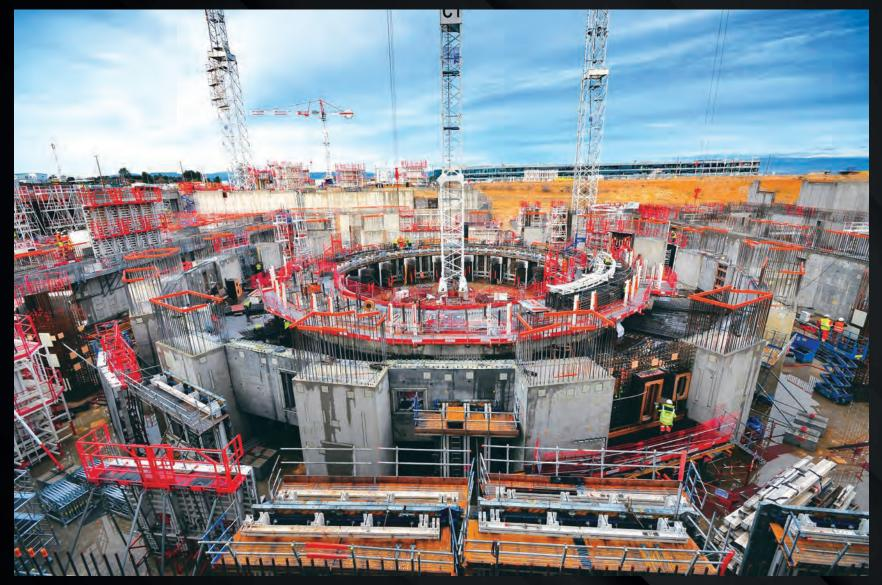
Around the three-metre-thick ITER bioshield in the centre is a wider circle formed by 18 giant columns that will rise 30 metres to provide structural support to the Tokamak Building.
