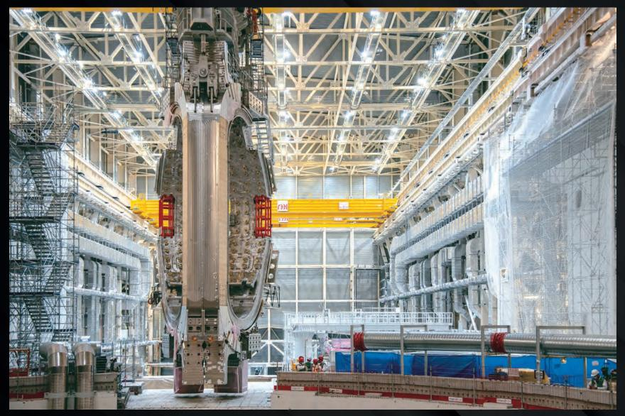
The first sector module—representing one-ninth of the torus-shaped vacuum vessel—is installed in the tokamak pit. Welded together, eight other similar assemblies will form the complete chamber and surrounding toroidal field coil superstructure.
