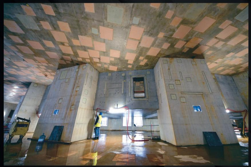
The cavernous spaces in the basement of the Tokamak Building will completely fill up with pipes, cables, feeders and busbars as the tokamak systems are installed. The equipment will be welded to the embedded plates that can be seen in the floor, walls and ceiling.
