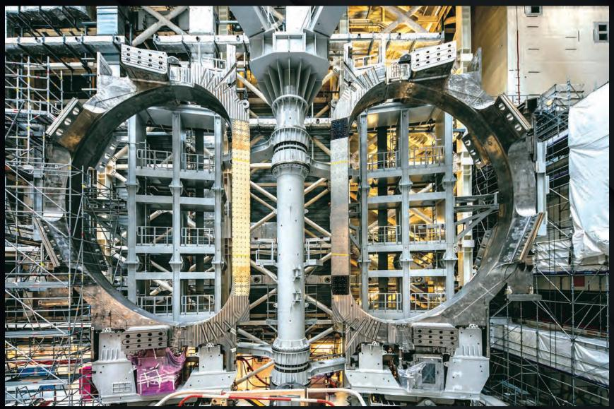
Displacement and dismantling operations have created a unique opportunity to photograph toroidal field coils in the wings of the tool without obstacle. Pictured are TF9 from Europe and TF8 from Japan.
