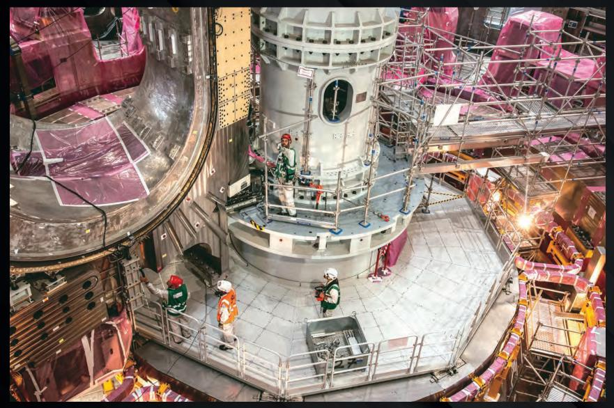
In order to repair the dimensional non-conformities in the vacuum vessel sectors and corrosion-induced cracks in the cooling pipes of the thermal shield panels, the decision is made to extract sector module #6 from the assembly pit for disassembly and repair. Vacuum vessel assembly activities must be temporarily halted.
