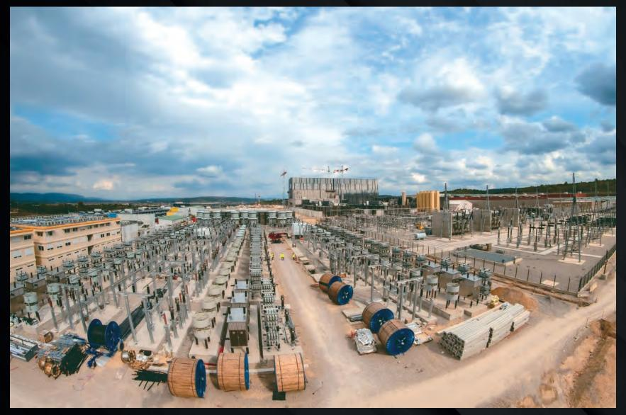
The reactive power compensation area accommodates reactors, capacitors, resistors and sensors that aim to smooth the flow of AC current both inside the ITER installation and in the immediate vicinity.
