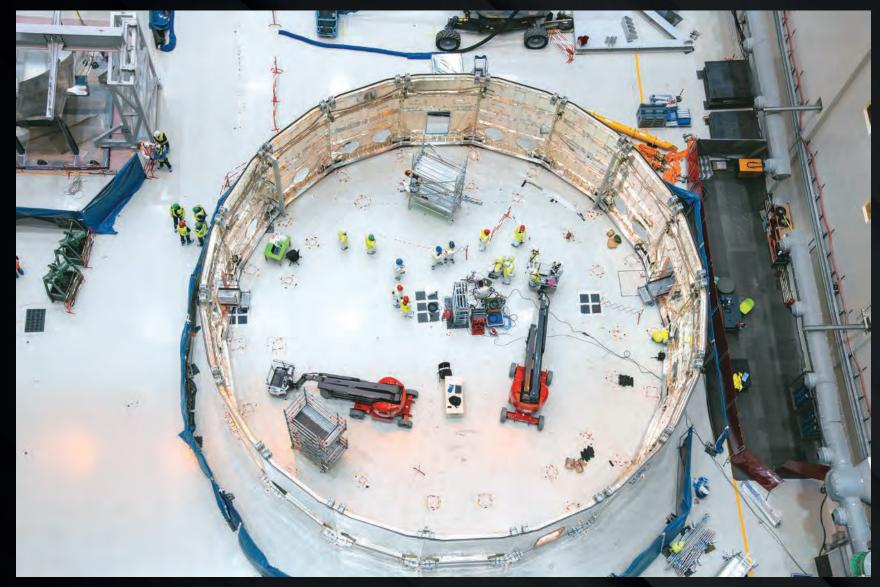
The lower cryostat thermal shield is being prepared for installation. The 10-millimetre-thin, 50-tonne component will fit inside the soup-dish-shaped depression of the cryostat base to form a heat barrier protecting the magnets at superconducting temperature. In the ITER Assembly Hall, all segments have been assembled.
