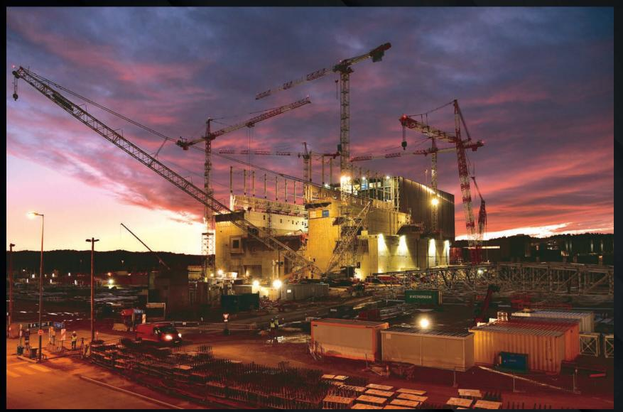
Over nine days in December, five pre-assembled modules for the roof of the crane hall are lifted into place. The complete roof structure—20 tall pillars and roof modules included—weighs approximately 2,000 tonnes.
