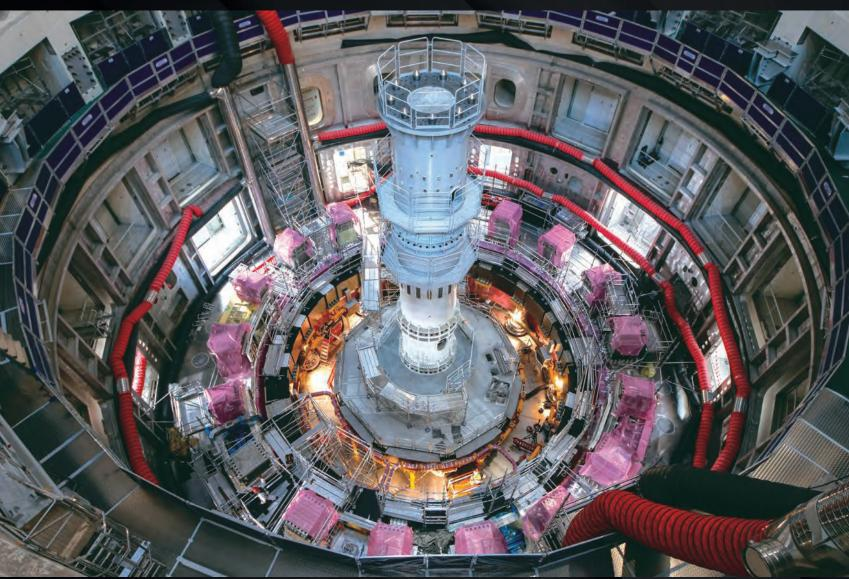
The first major machine components are in place at the bottom of the tokamak pit—the base and lower cylinder of the cryostat, the first two poloidal field coil magnets, and 18 supports for the toroidal field magnets. The first vacuum vessel sector will join them next year.
