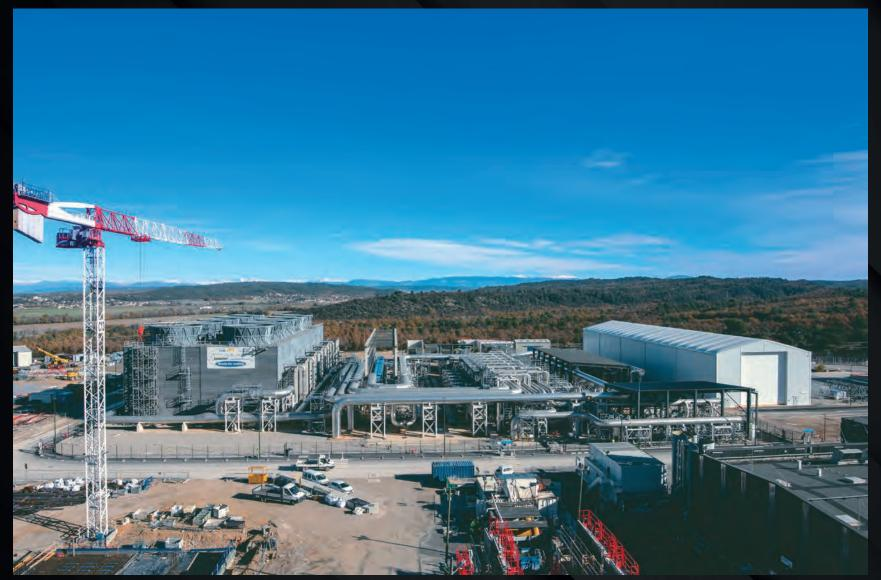
The heat rejection system is the final cooling loop of the ITER installation, ultimately dissipating the heat load generated during operation. The necessary infrastructure is concentrated in a 6,000-square-metre area (background) that comprises hot and cold cooling water basins, powerful pumps, heat exchangers, and an induced-draft cooling tower with ten individual cells.
