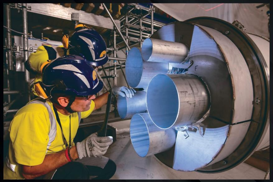
Cryolines travel back and forth between the cryoplant, where cooling fluids are produced, and the Tokamak Building. One section of cryoline can host up to six or seven "process pipes," each devoted to a specific fluid, flow direction or function.
