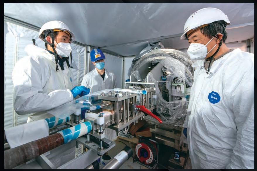
Deep in the basement of the Tokamak Building, trained specialists are assembling the first superconducting feeder joints to connect high-current busbars. This highly technical operation must be repeated approximately 300 times.
