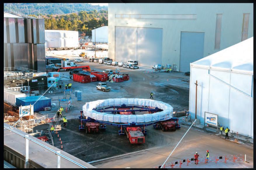
Poloidal field coil PF2 measures 17 metres in diameter and weighs just over 200 tonnes. In December, it was moved to temporary storage—the second of four ring-shaped coils to exit the on-site European manufacturing facility.
