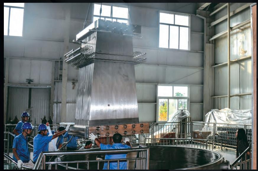
Eighteen pillar-like gravity supports will be bolted to the cryostat base to support the toroidal field coil structure, shouldering the dead weight of the tightly integrated magnet system while withstanding the displacement of the coils during cooldown and operation. The cooling system of this unit is about to undergo helium leak testing.
