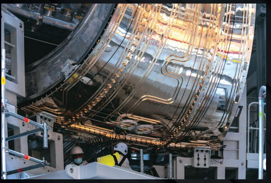
Once suspended vertically in tooling, a vacuum vessel sector is paired with its thermal shield (visible in this picture) and two toroidal field coils. The result is a "vacuum vessel sector module," ready for transfer into the tokamak pit.
