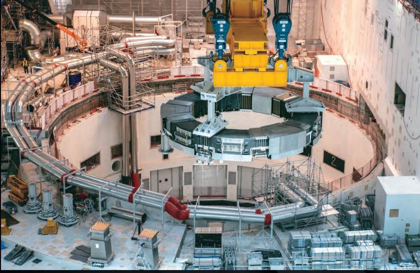
The installation of the first magnet, 330-tonne poloidal field coil PF6, is a major assembly milestone achieved in April.
