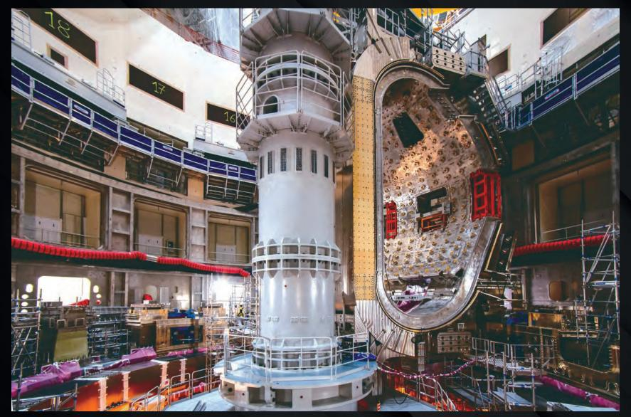
In the last phase of the lift and installation, the sector module is suspended only 50 centimetres above its supports in the assembly pit, as the assembly team carries out final metrology. Team coordination, the overhead crane's lifting capacity, and rigging maneuverability were all tested successfully during this first-of-a-kind operation.
