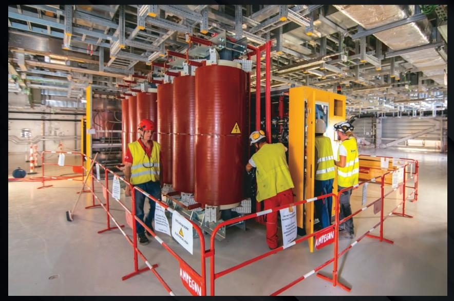
A high-voltage power supply system is installed in the Radio Frequency Building for the electron cyclotron resonance heating system, one of three auxiliary heating systems on ITER.
