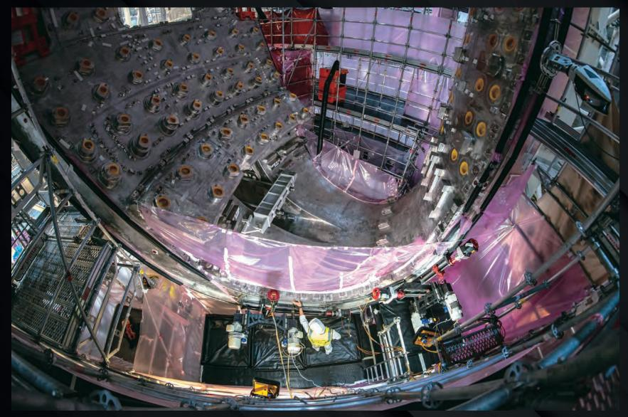
The geometry of the outer shell field joints—where sectors are to be welded together—must be restored to nominal so that the access and operation of the bespoke automated welding tools in the tokamak pit is not compromised. Two sectors are being repaired in vertical tooling; a third, sector #8, will be repaired in a horizontal position.
